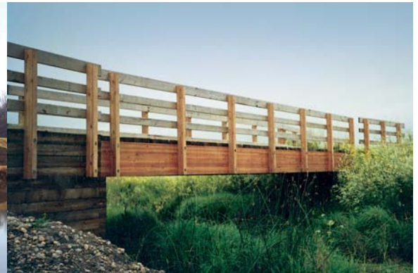
Pre-fabricated Timber Bridge
