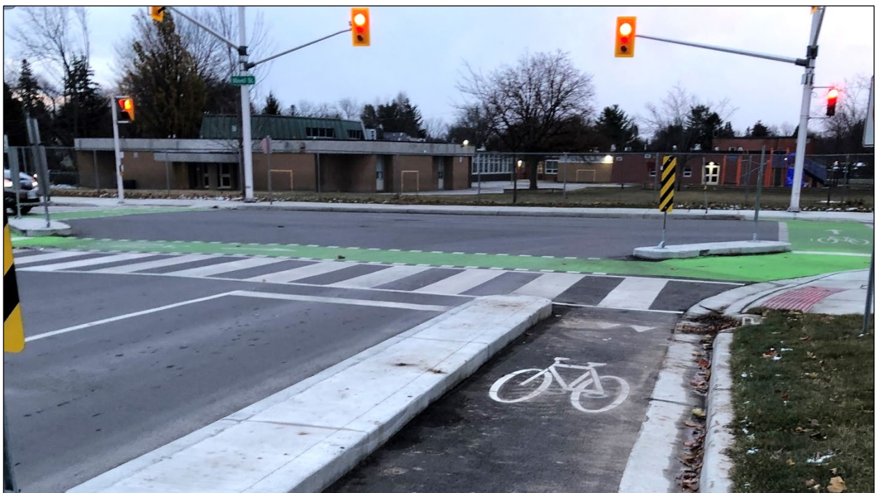
Cycling protected intersection with a corner refuge island – London, Ontario (Arcadis photo)
