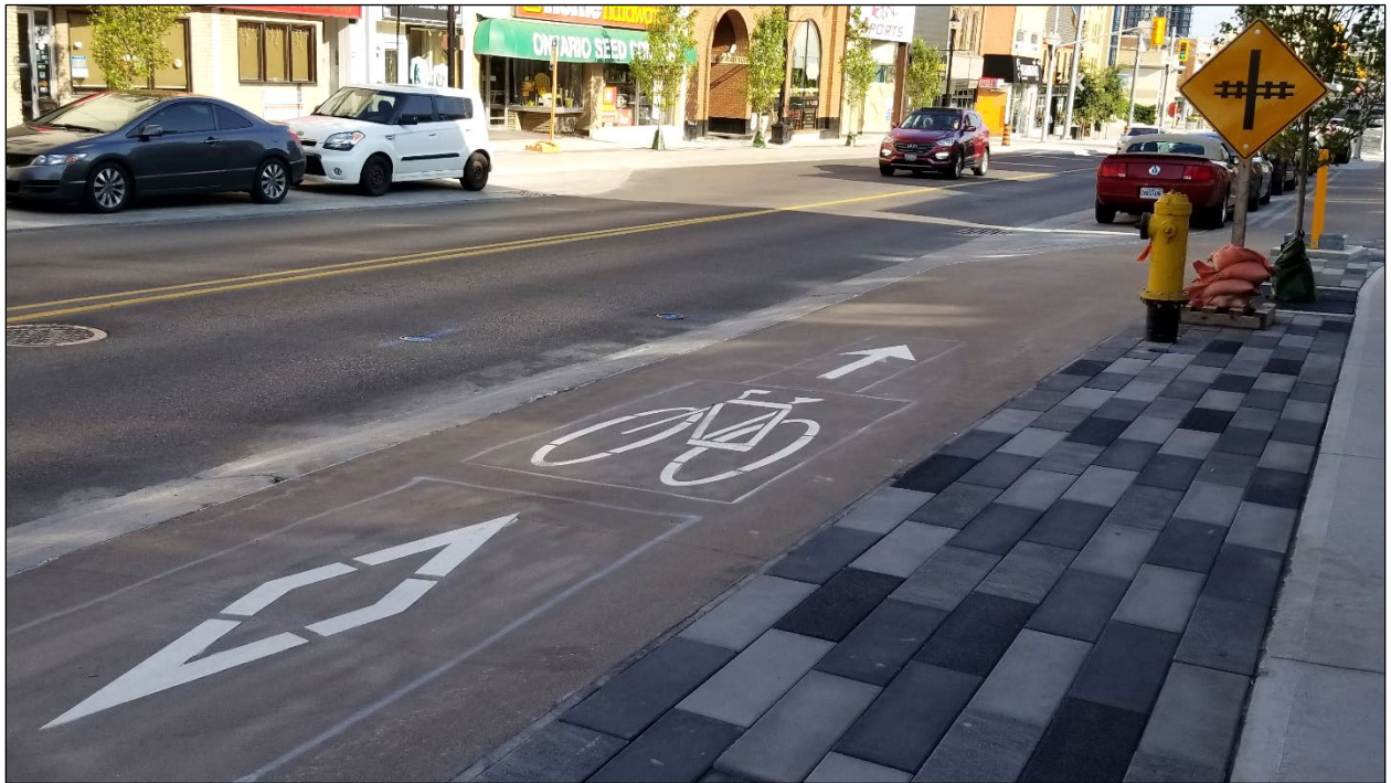
Mountable curb separating a one-way cycle track – Waterloo, Ontario (Arcadis photo)
