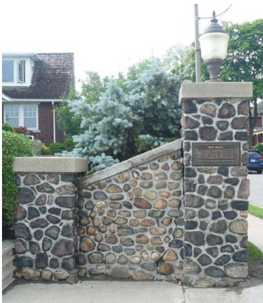
Existing Heritage Feature
