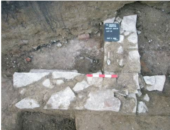
An example of a stone foundation
