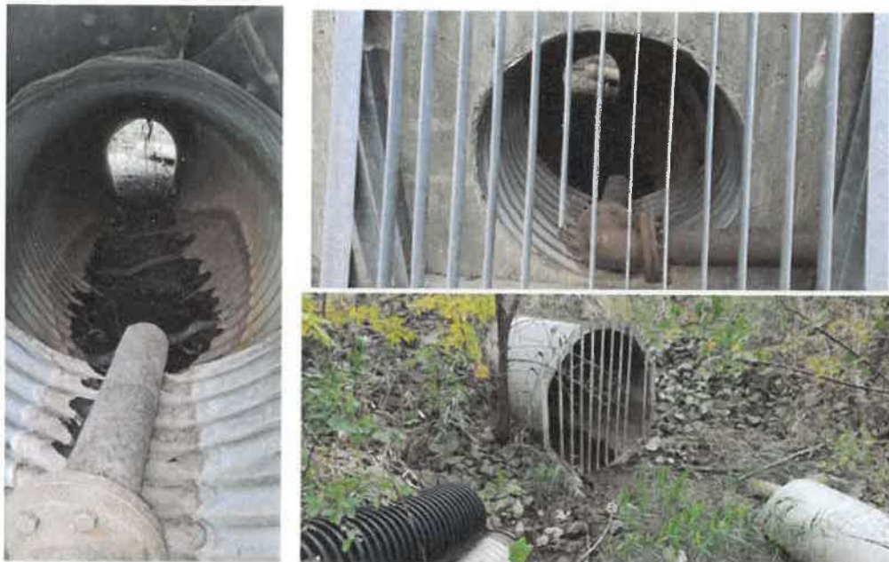
Photograph 2 – Current Central Pond Outlet
