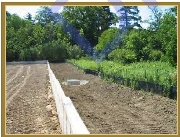
Plate 6. Stand-alone continuous concrete wall used to exclude salamander species installed as pre-cast forms (photo credit: Steven Roorda).
