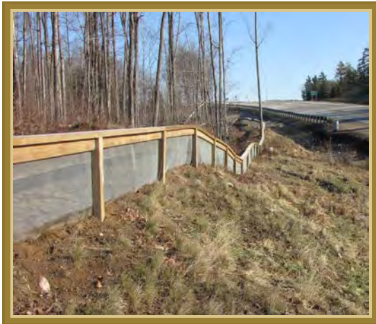
Plate 3. Example of a galvanized mesh fencing used for the long-term exclusion of snakes and turtles from the adjacent highway (photo credit: Megan Bonenfant).
