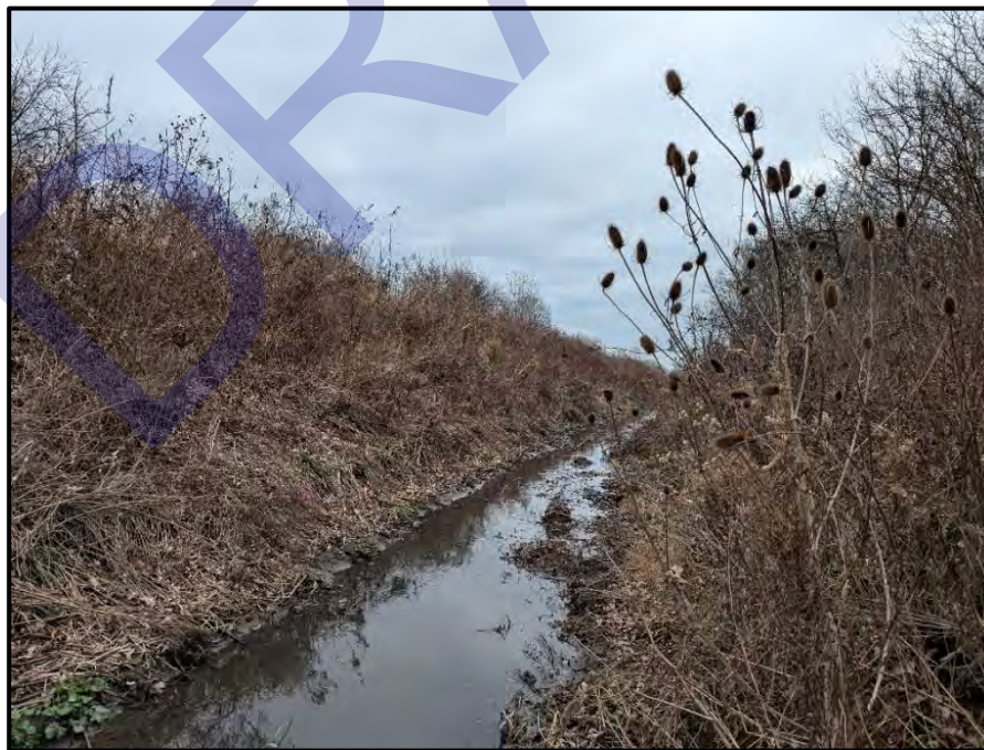
Picture 7: Hawkins Drain, looking east, during December 2024 field investigations.
