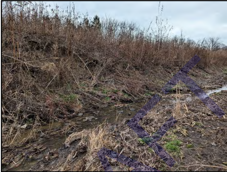
Picture 6: Hawkins drain, looking east, during December 2024 field investigations.
