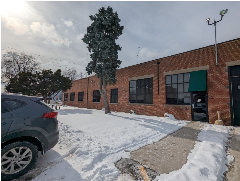
Photos 27 & 28: Views of the east elevation of the structure. (MHBC, 2025)
