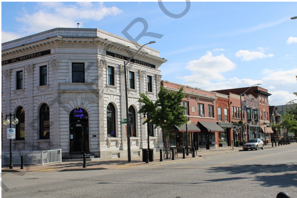
Figure 35: View of the former Bank of Montreal, 2024
