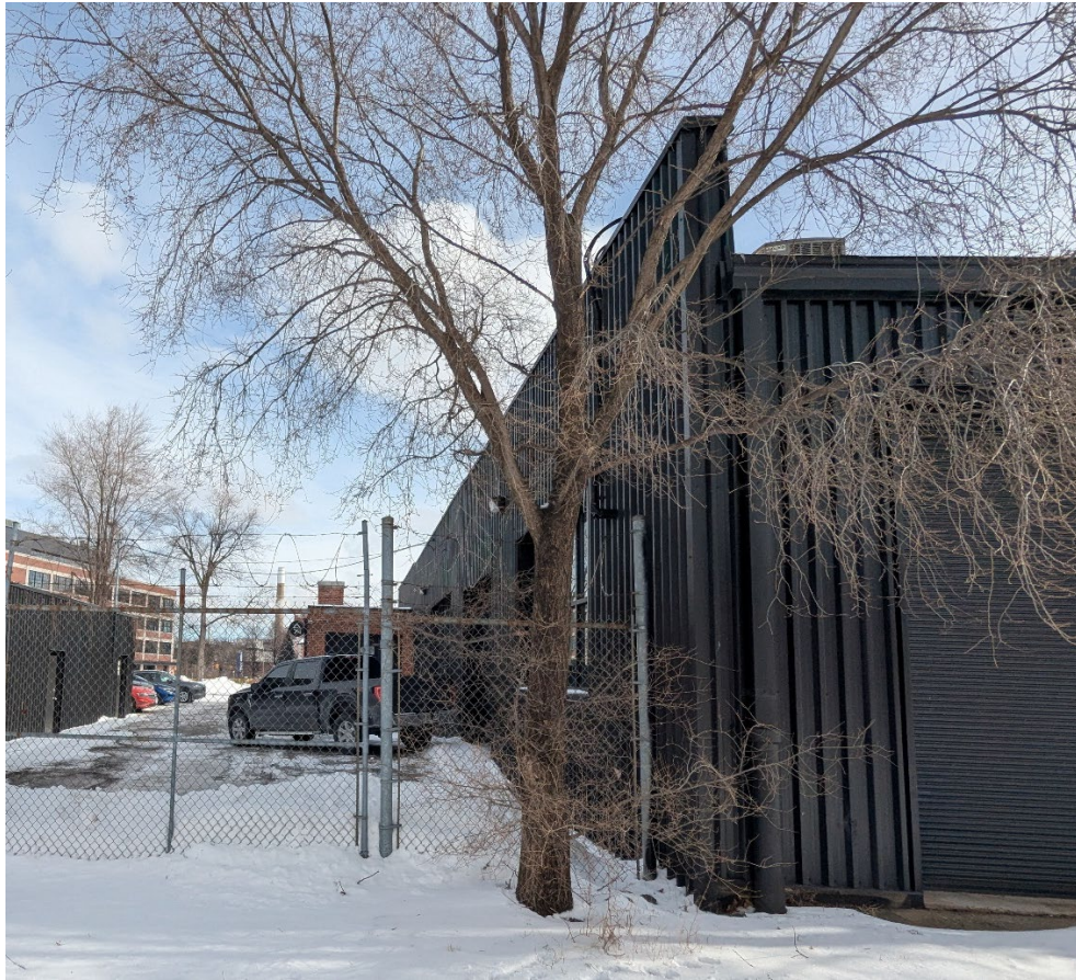
Photos 31-33: Views of the north elevation of the structure. (MHBC, 2025)
