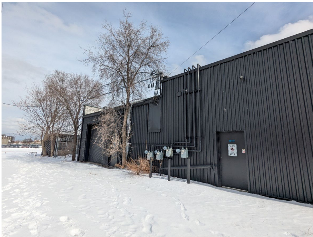
Photos 29 & 30: Views of the west elevation of the structure. (MHBC, 2025)
