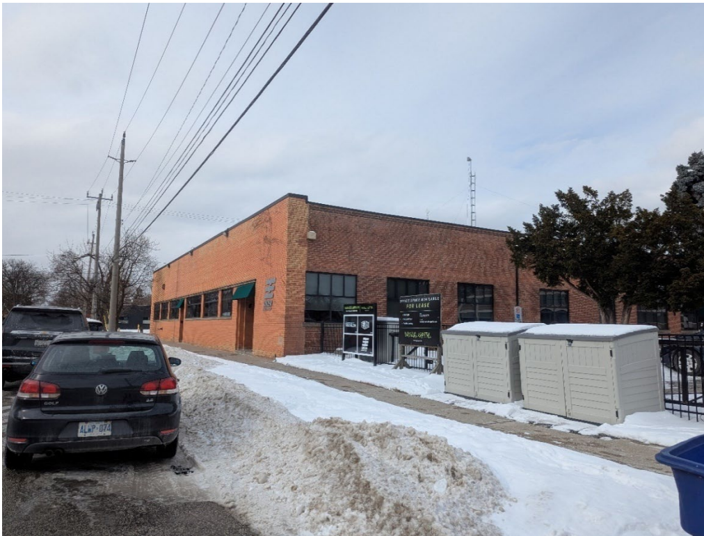
Photos 23 & 24: Views of the south (principal) elevation of the structure on the subject property. (MHBC, 2025)
