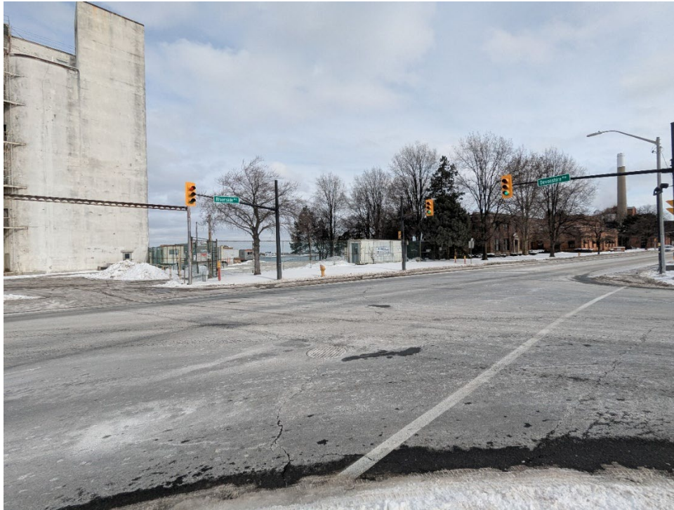
Photo 3: Looking east from the intersection of Devonshire Road and Riverside Drive East. (MHBC, 2025)
