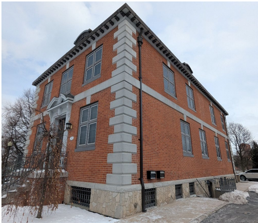
Photo 22: View of the Walkerville Town Hall. (MHBC, 2025)
