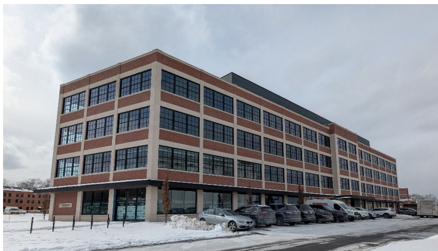
Photo 15: View of the north and east elevations of the Walker Power Building. (MHBC, 2025)
