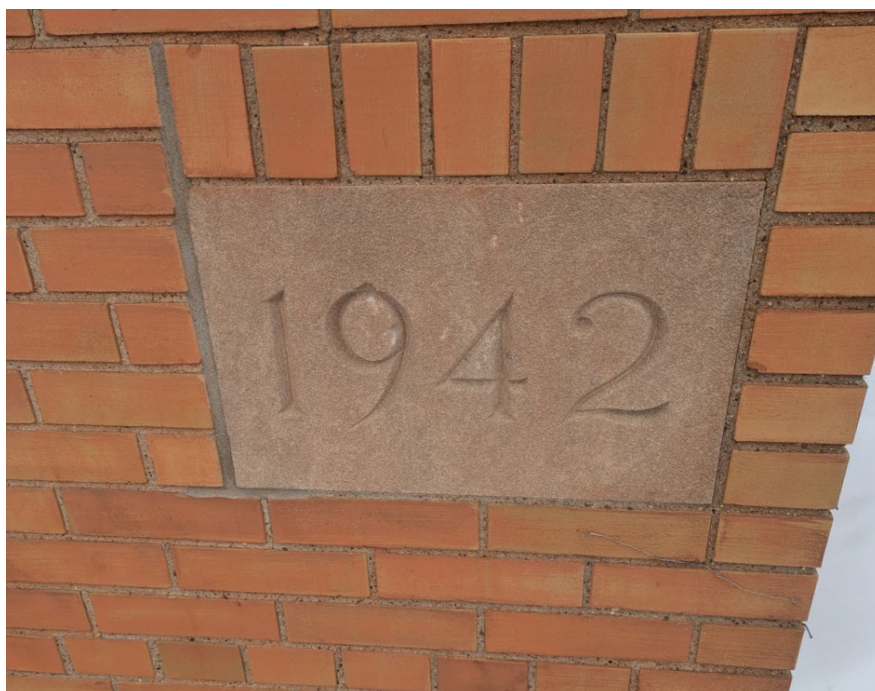
Figure 20: View of the date stone on the south façade of the existing building. (MHBC, 2025)
