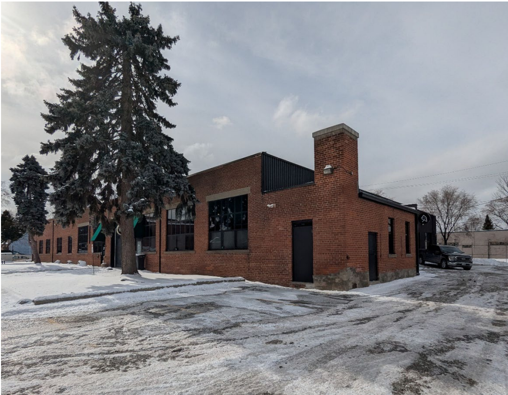
Photos 25 & 26: Views of the east elevation of the structure. (MHBC, 2025)
