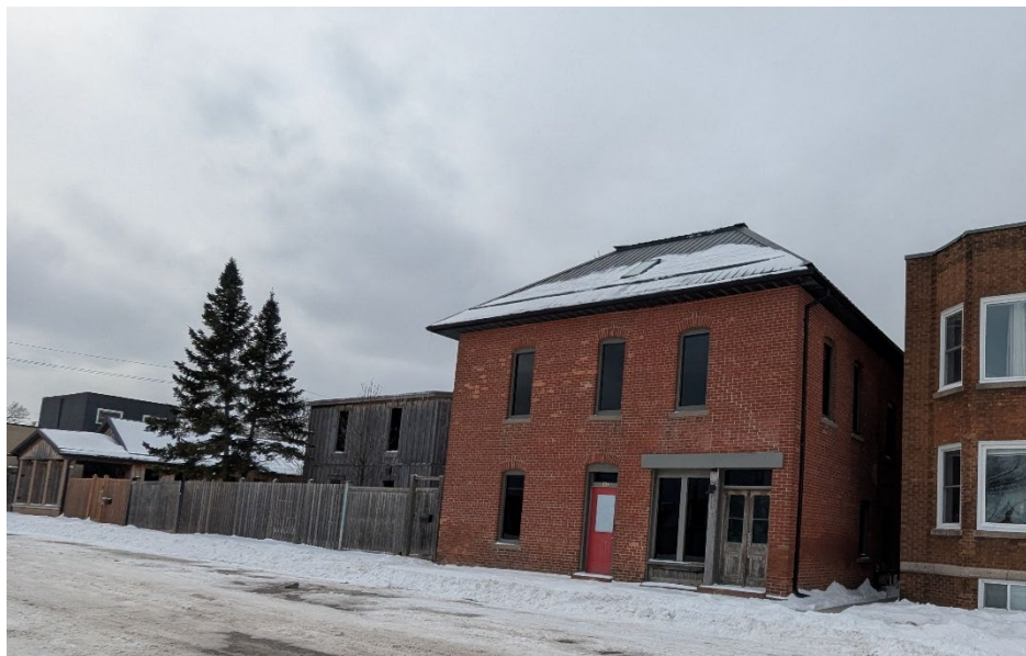
Photo 17: View of the principal elevation of 341-343 Chilver Road. (MHBC, 2025)
