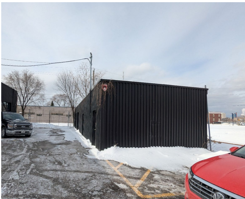
Photos 34 & 35: Views of the accessory structure. (MHBC, 2025)
