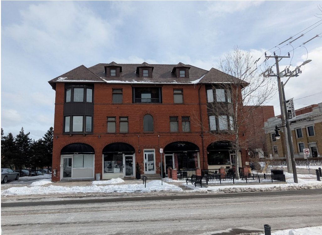
Photo 21: View of the principal (west) elevation of the Crown Inn. (MHBC, 2025)
