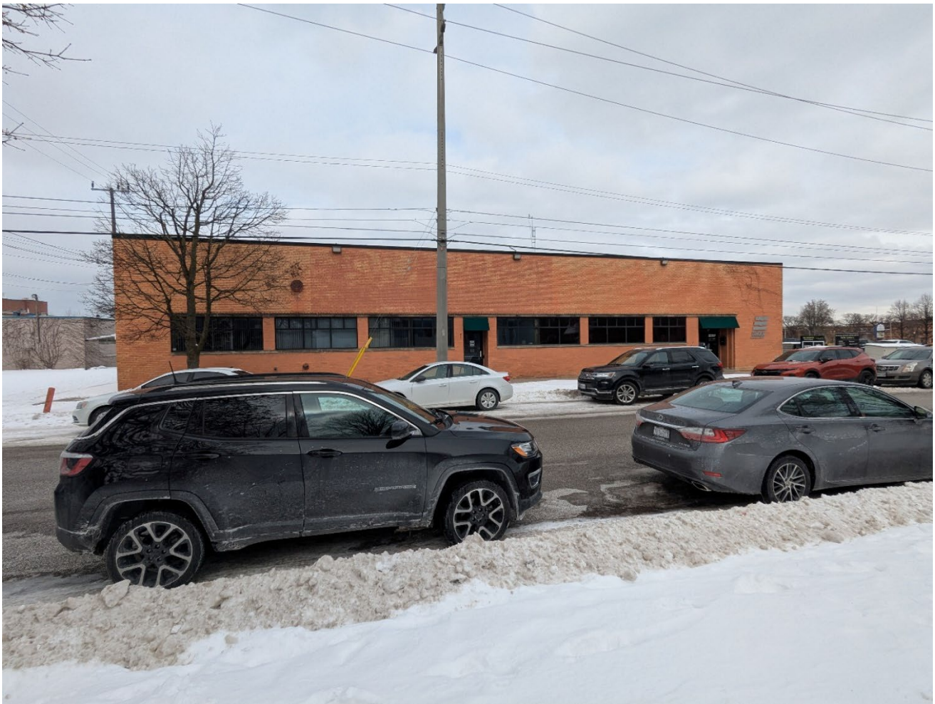
Photo 1: View of the principal elevation of the subject property. (MHBC, 2025)
