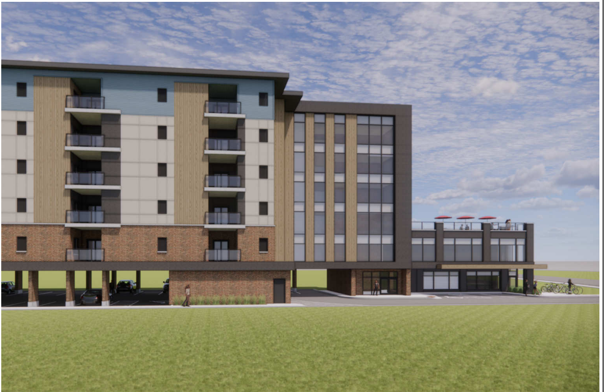
VIEW OF WEST FACING ENTRY
