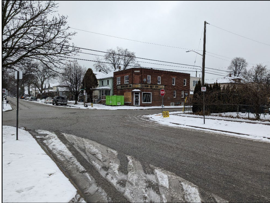
Figure 1b – Site Street View (Source: Pillon Abbs Inc.)
