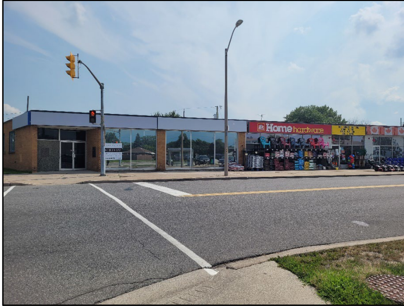
Photos 2 – South (Source: Pillon Abbs Inc.)
