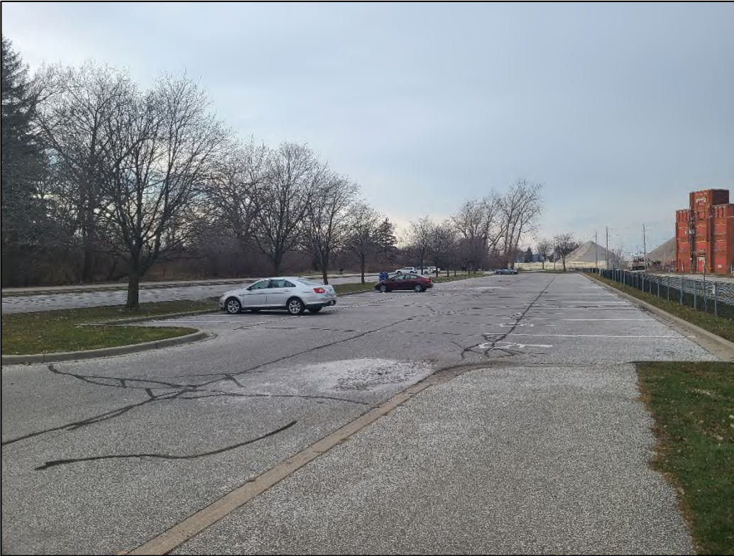
PHOTO 1: PARKING LOT – LOOKING WEST FROM FLORENCE AVE.
