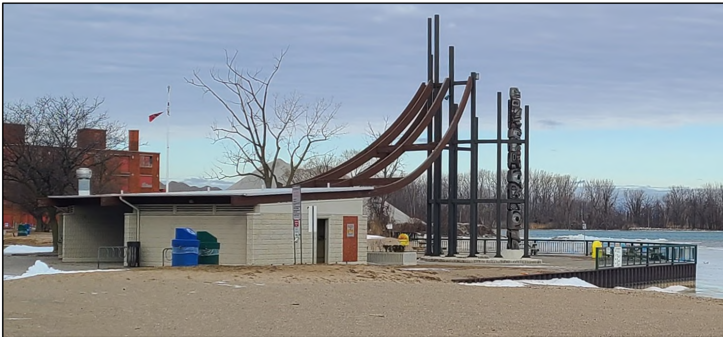
MAIN FACILITIES BUILDING (LOOKING WEST TOWARD THE EAST BUILDING)
