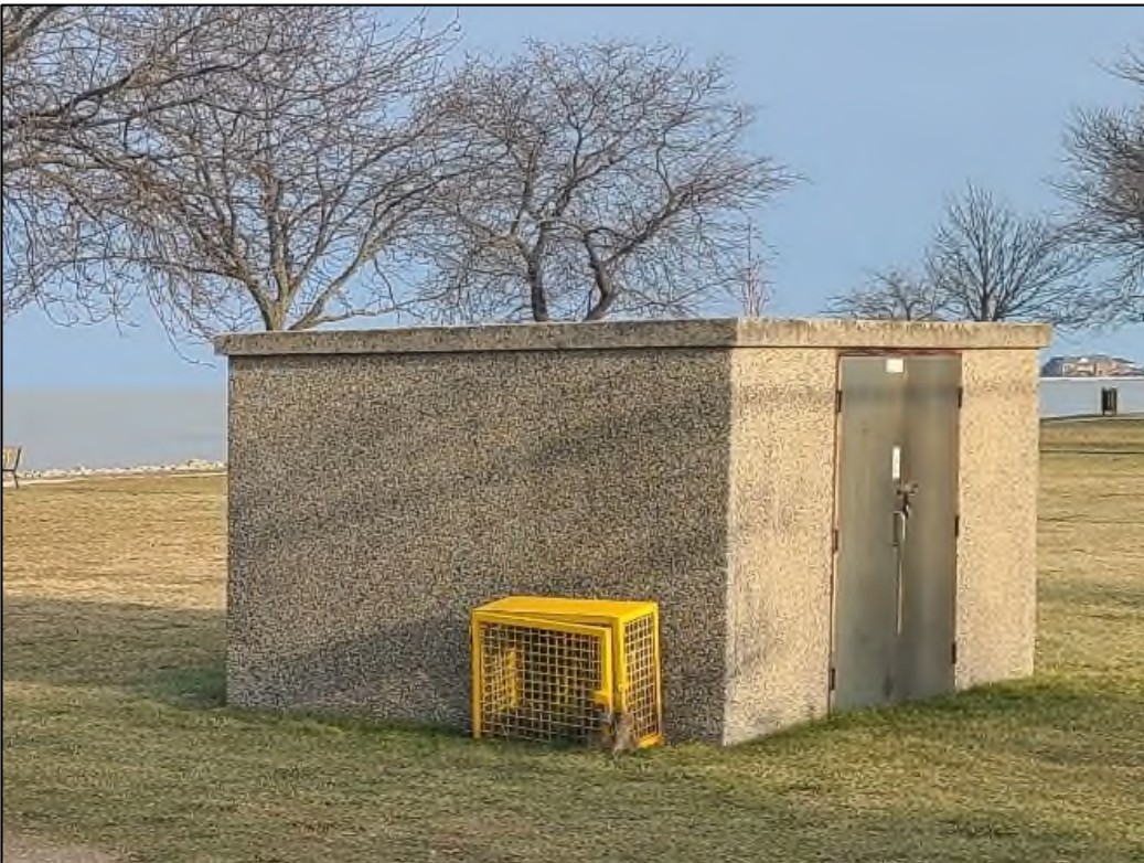
PPHOTO 14: STORAGE BUILDING IN GANATCHIO PARK
