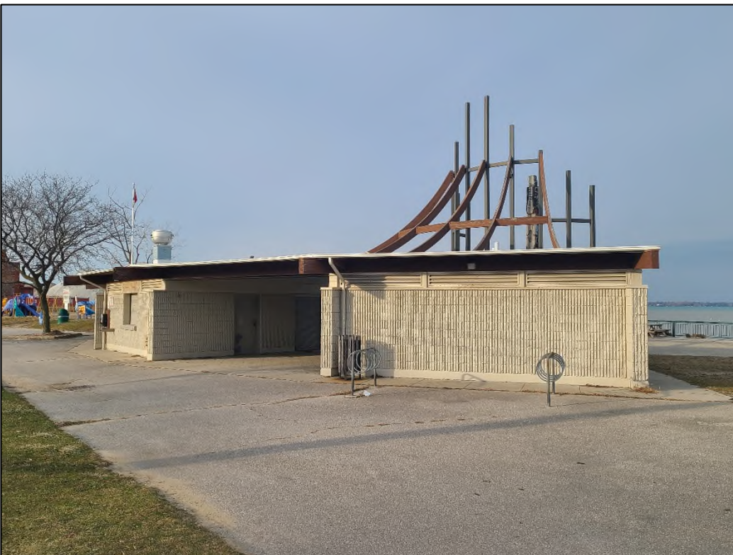
PHOTO 4: MAIN FACILITIES / WASHROOM BUILDING (BACK OF BUILDING)
