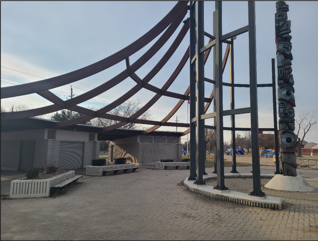
PHOTO 3: MAIN FACILITIES / WASHROOM BUILDING (FRONT OF BUILDING) & TOTEM POLE
