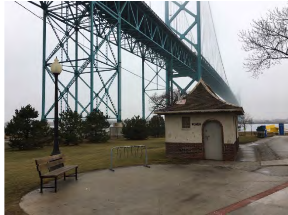
Photo 22: View of Parcel 2 Study Area Illustrating Existing Municipal Building, facing northwest
