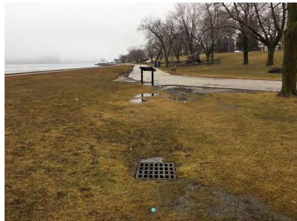
Photo 24: View of Parcel 2 Study Area Illustrating Subsurface Municipal Infrastructure and Area of Land Reclamation, facing east-northeast
