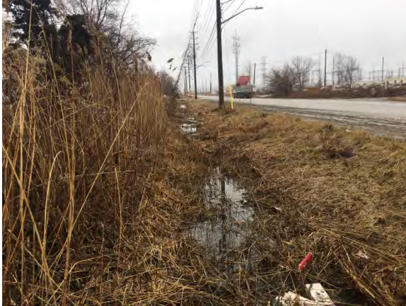
Photo 9: View of Parcel 1 Study Area Illustrating Disturbed Drainage Ditch, facing south-southwest
