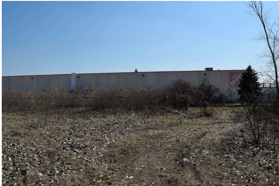
IMAGE 4: VIEW OF PREVIOUSLY DISTURBED AREA LOCATED AT THE REAR OF THE EXISTING BUILDINGS, FACING SOUTH-SOUTHWEST
