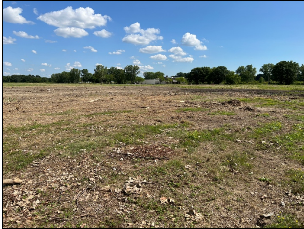
Image 3: Showing Disturbed Conditions of Test Pitting Survey
