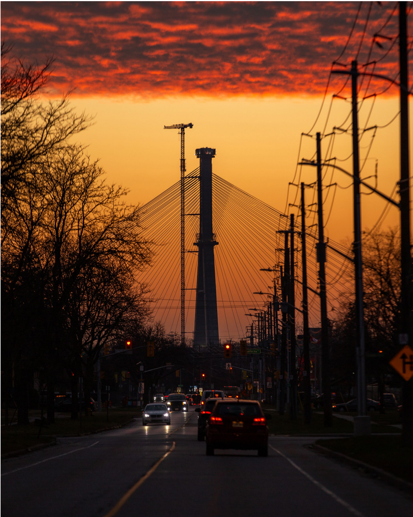
Construction of the Gordie Howe International Bridge.
