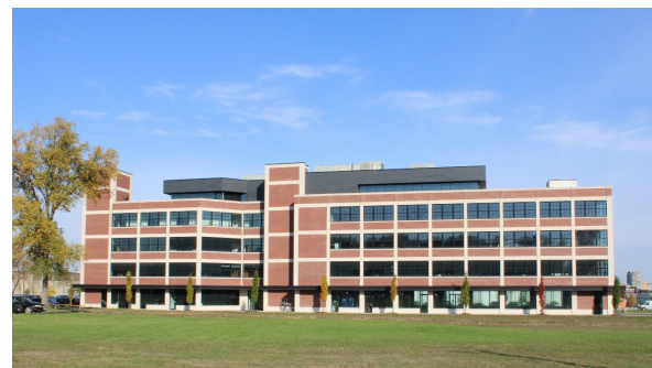
Figure 29: The results of a recent adaptive re-use project at 325 Devonshire Road, Fall 2023
