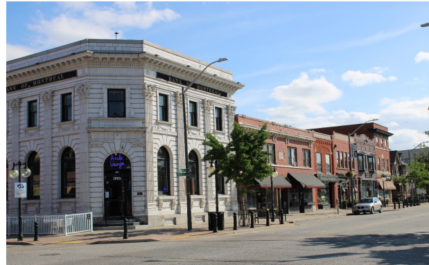
Figure 36: View of the former Bank of Montreal, 2024
