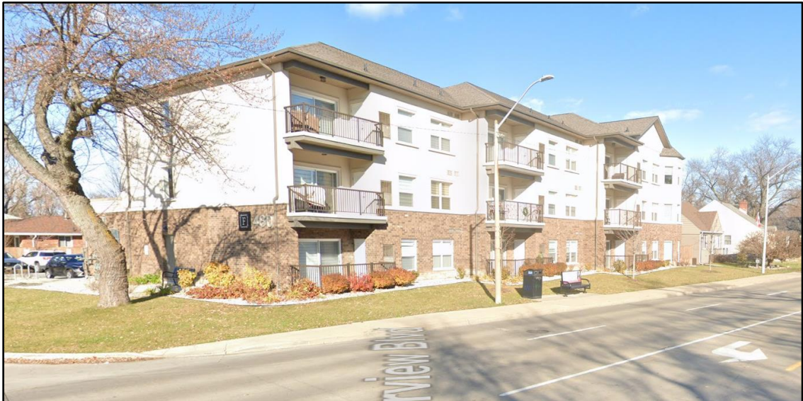
Wyandotte Street East (Fairview Blvd intersection) – low-rise multiple dwelling
