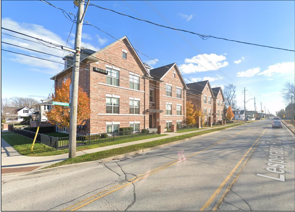
Lesperance Road (Town of Tecumseh)- Low rise multiple dwellings
