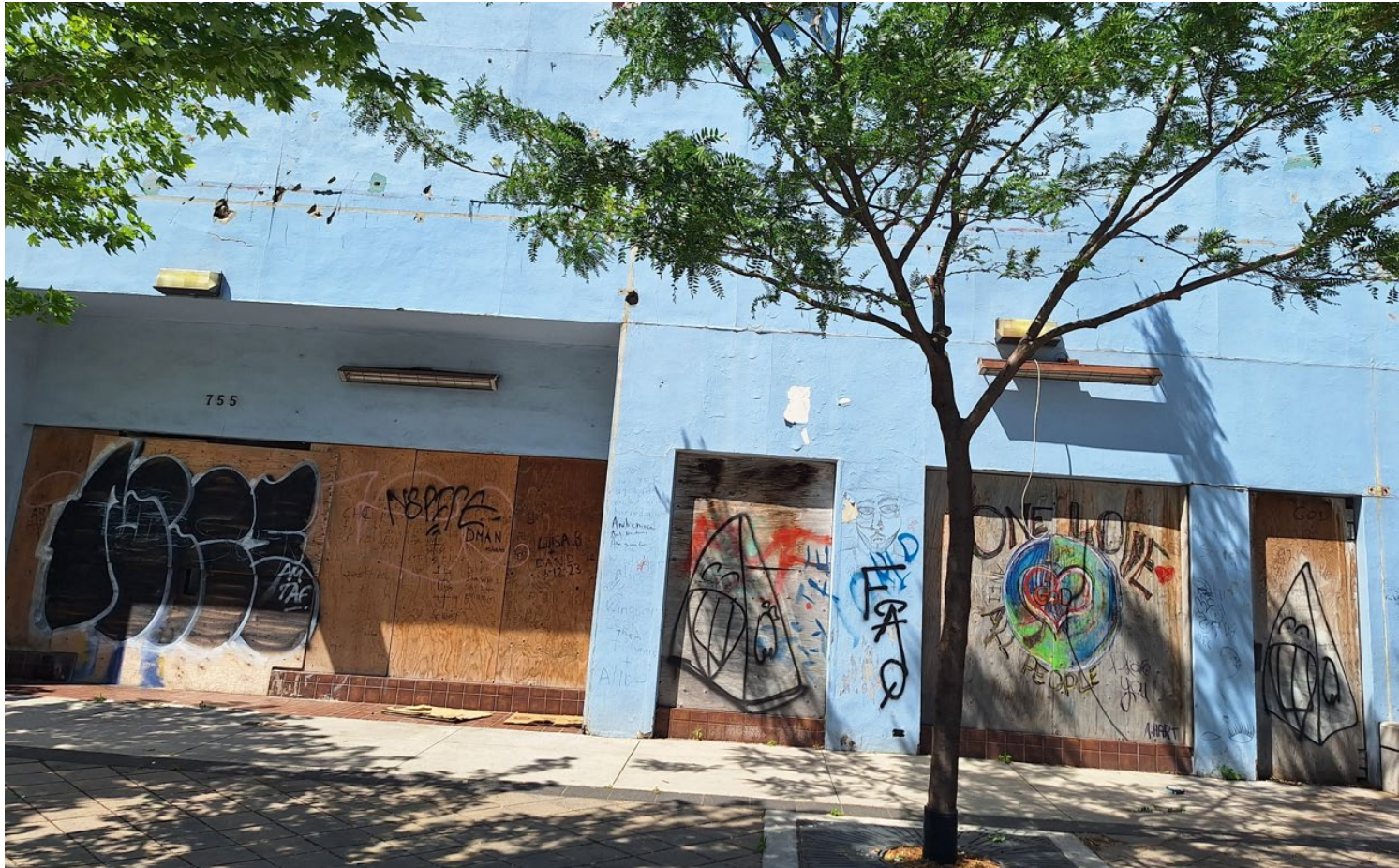
EAST (FRONT) SIDE OF BUILDING (CLOSE UP) FACING OUELLETTE AVE
