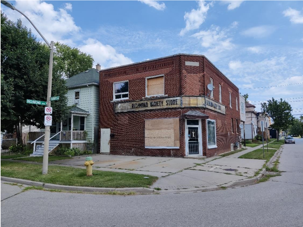
View northeast towards the subject parcel.
