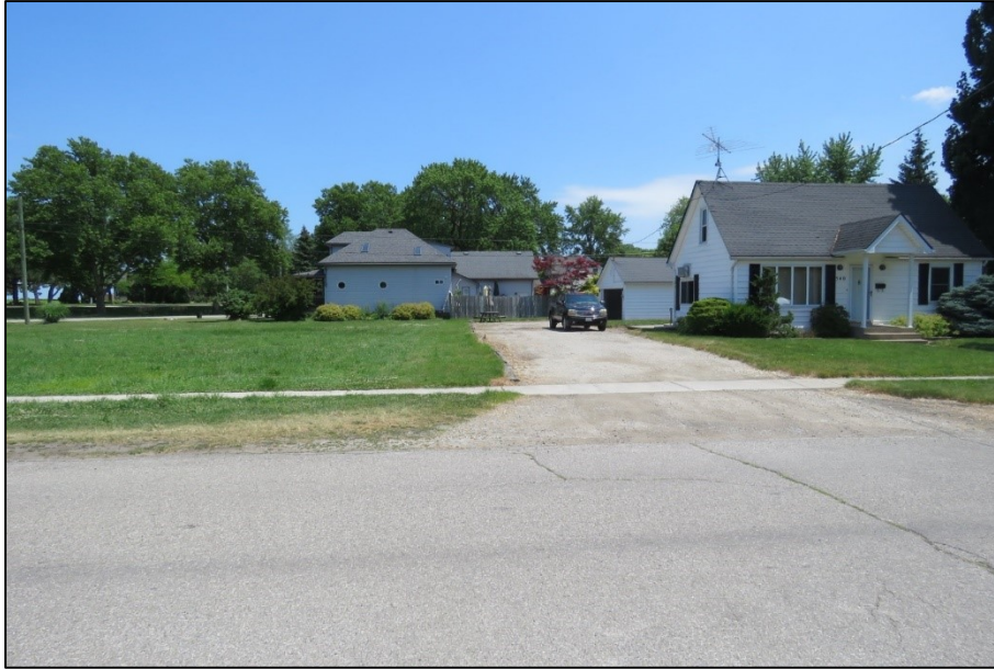
Figure 1 - Looking east towards east/west alley from Clover Street (540 Clover Street on right)
