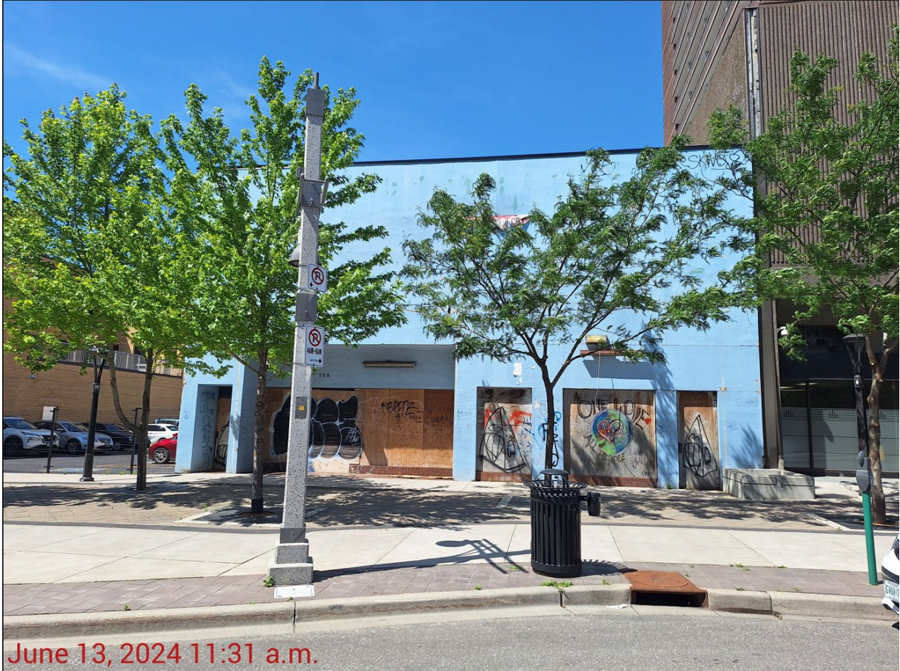
EAST (FRONT) SIDE OF BUILDING FACING OUELLETTE AVE
