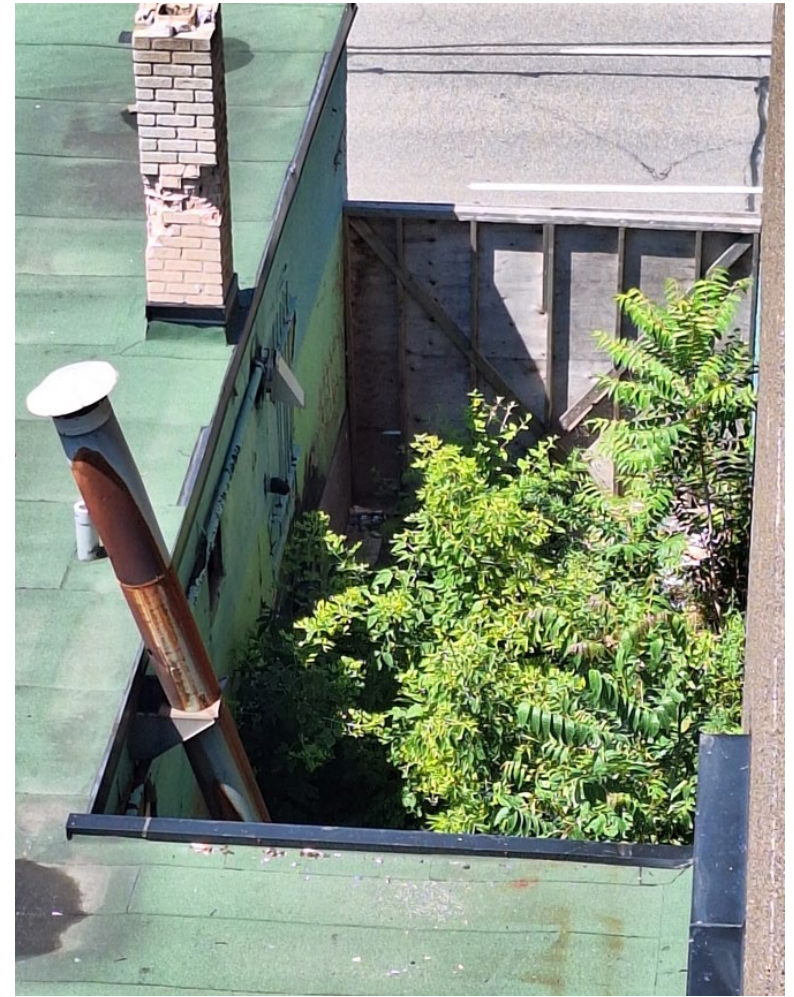
HOLE IN ROOF; DETERIORATING CHIMNEY; OVERGROWN SCRUB TREES
