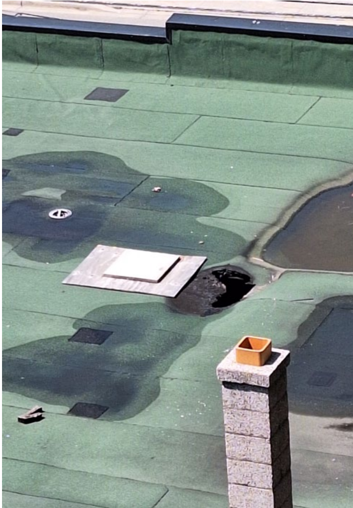
HOLE IN ROOF; DETERIORATING CHIMNEY; OVERGROWN SCRUB TREES
