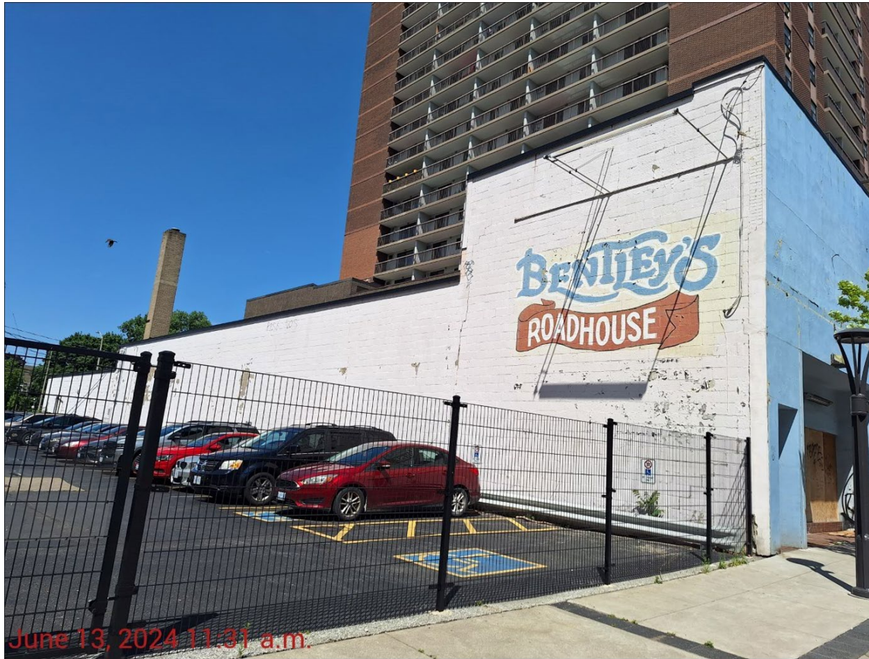
SOUTH SIDE OF BUILDING
