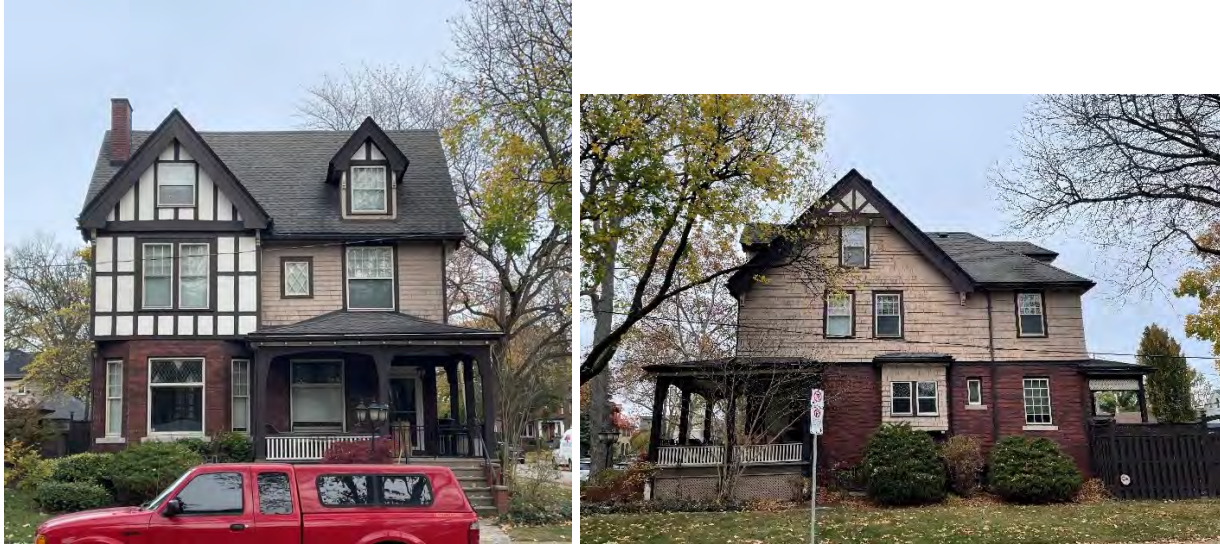
Front (west-facing) and side (south-facing) views of the property.
