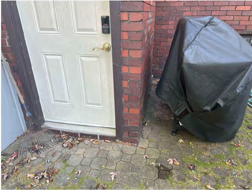
Waterproof side wall of grade entrance
