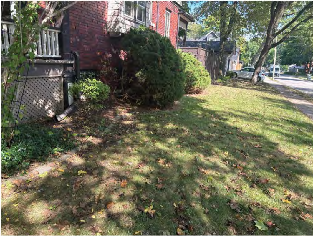
South wall - entire wall
