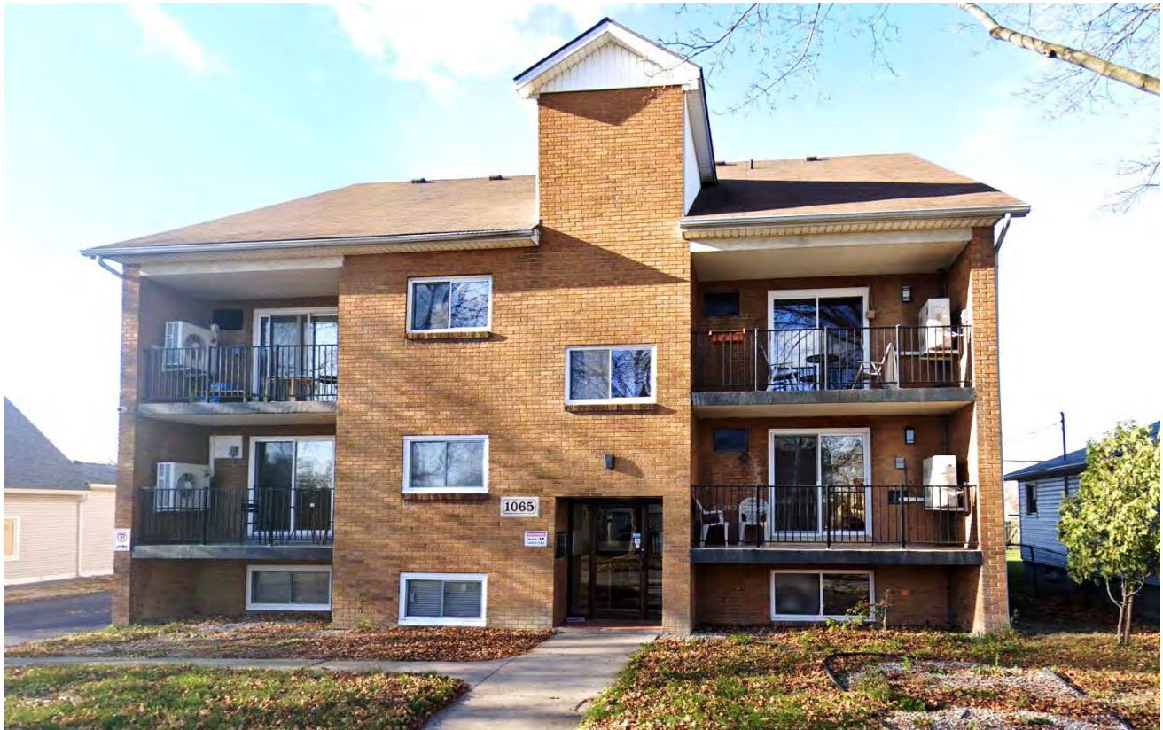
FIGURE 10: 1065 CALIFORNIA (ACROSS CALIFORNIA – 2.5 STOREY MULTI-UNIT BLDG)
