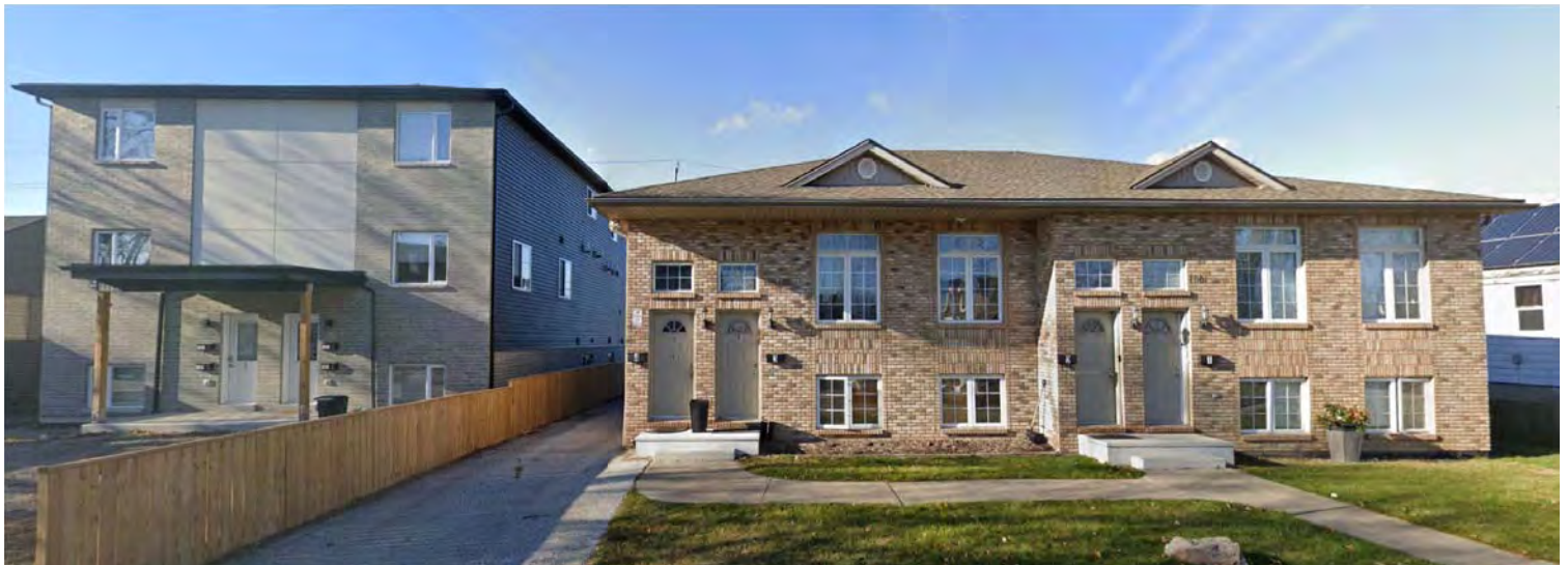
FIGURE 12: 1081 AND 1091 CALIFORNIA AVE (SOUTH-2 & 2.5 STOREY MULTI-UNIT BLDG)
