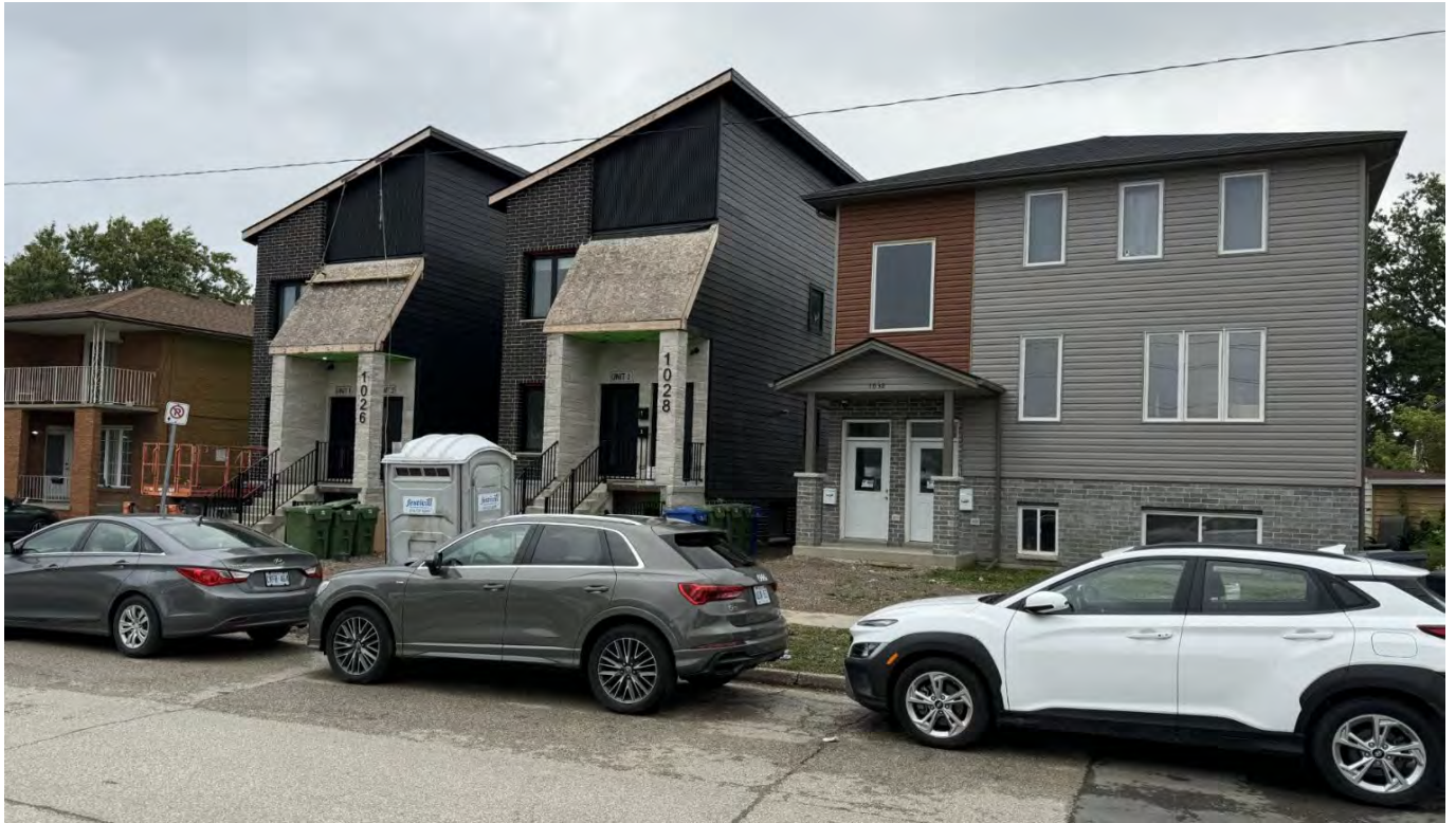
FIGURE 11: 1026 CALIFORNIA and 1028 CALIFORNIA AVE
