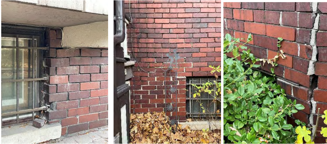
Photos of the brick foundation walls (taken November 13, 2024)
