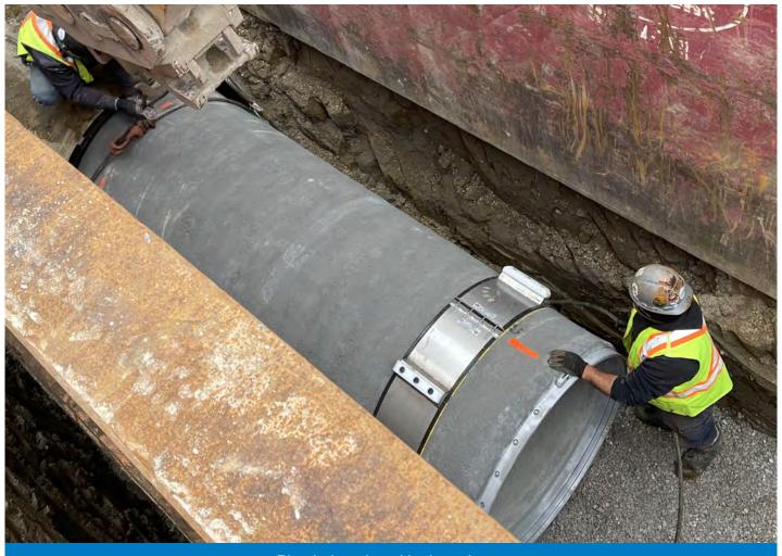
Pipe being placed in the caisson
