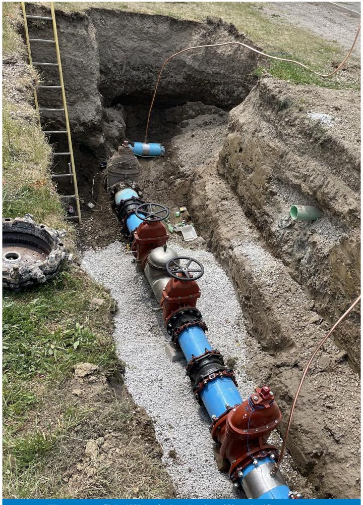
Water source to fill the 1050 mm feedermain using a 250 mm backflow preventer
