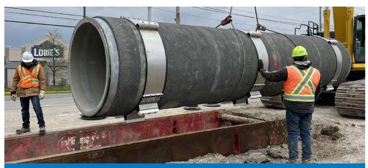
Pipe with spacers ready to be placed in the caisson
