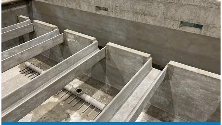
Filter Bed Rehabilitation (Phase 4): Filter #6 concrete surface waterproofing
