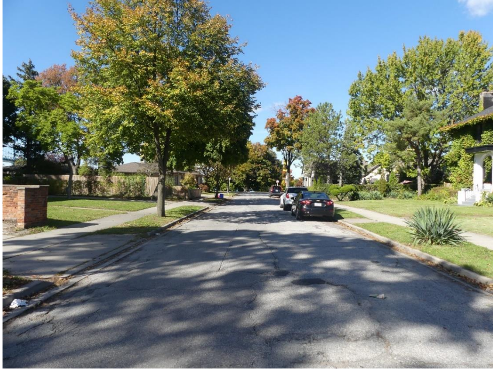
View along California Avenue looking north
