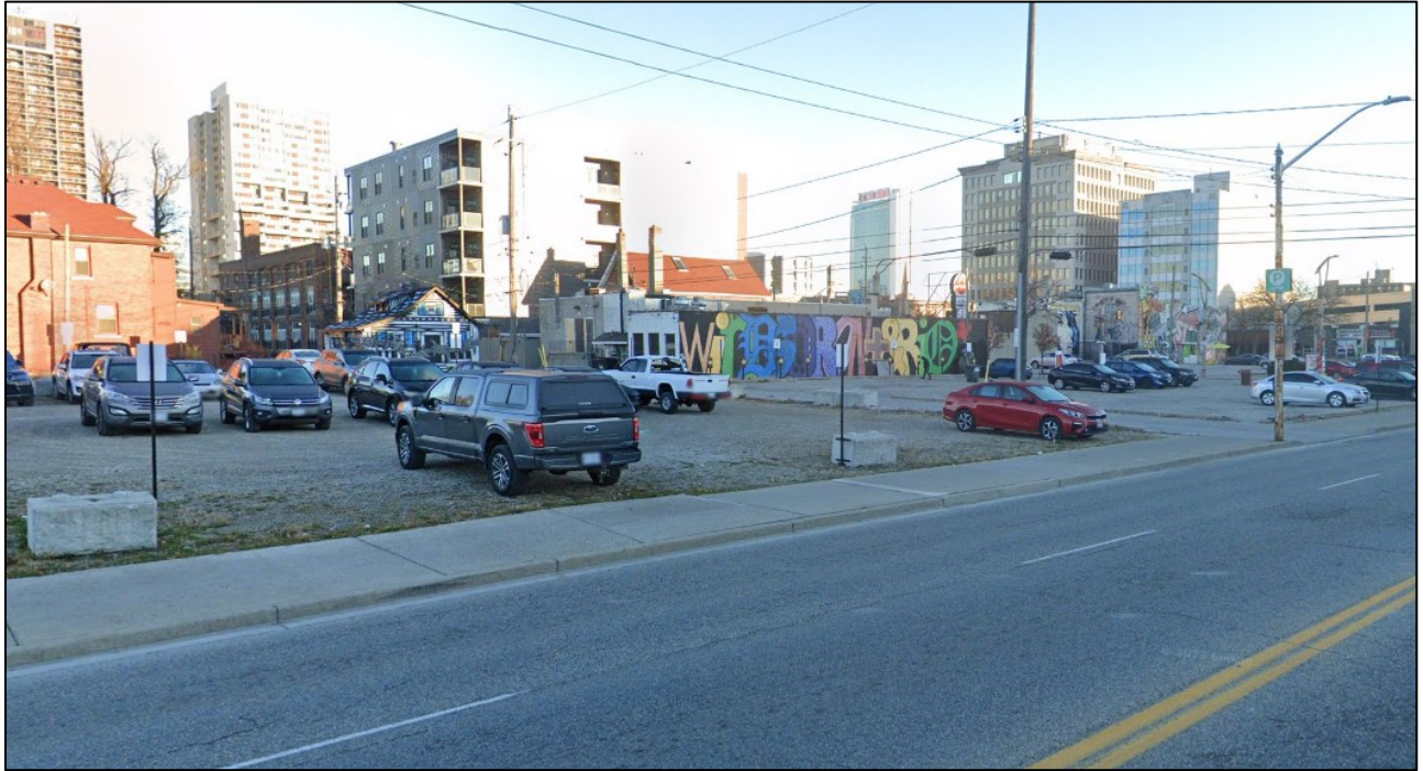
Figure 3 - Looking northeast towards alley from Wyandotte St W (170 Wyandotte St W on left)
