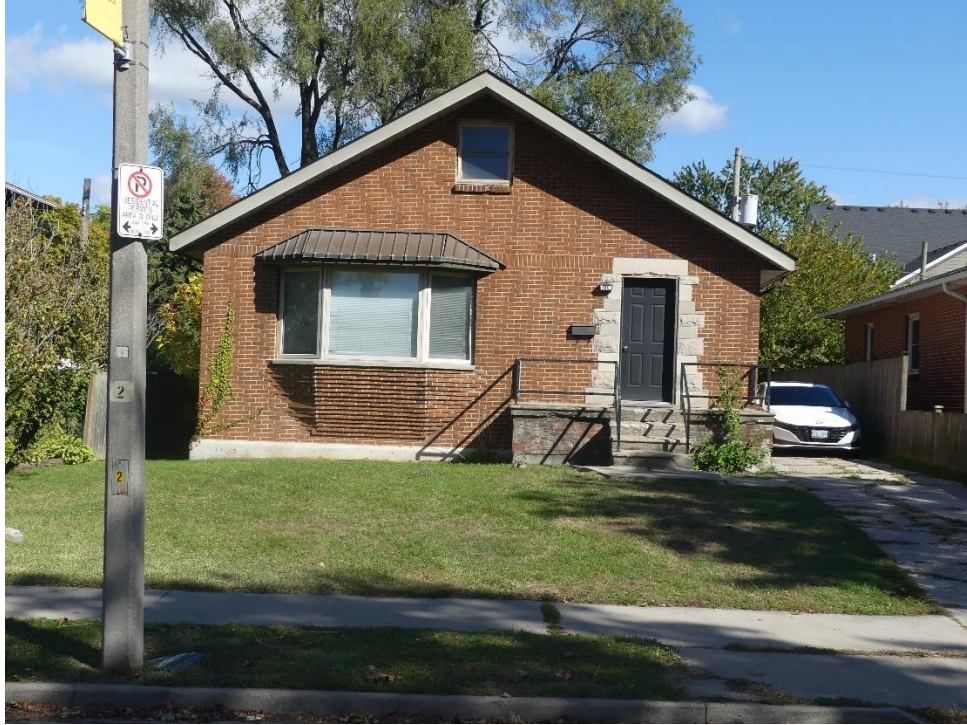
View of the subject parcel, looking east
