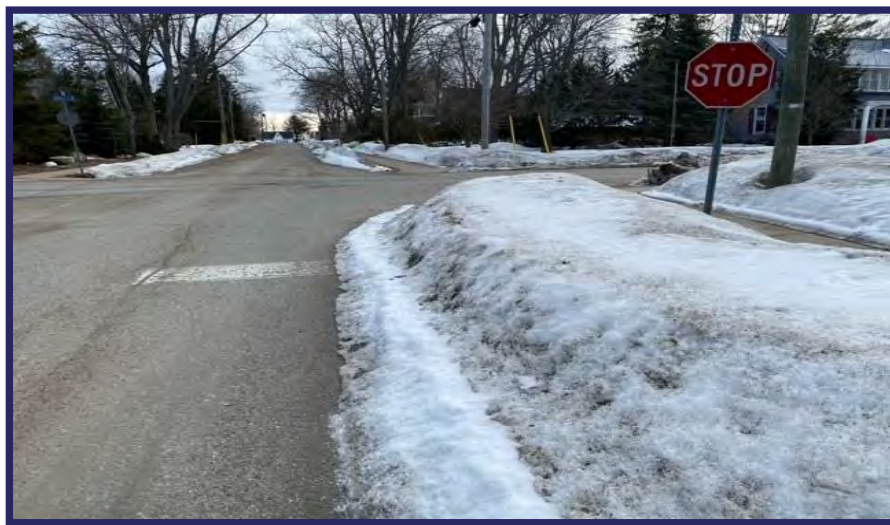
Photo: snow-narrowed roadway.
