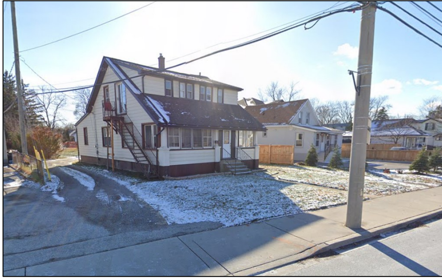
Figure 3 - Looking southwest towards 4461 Wyandotte Street East
