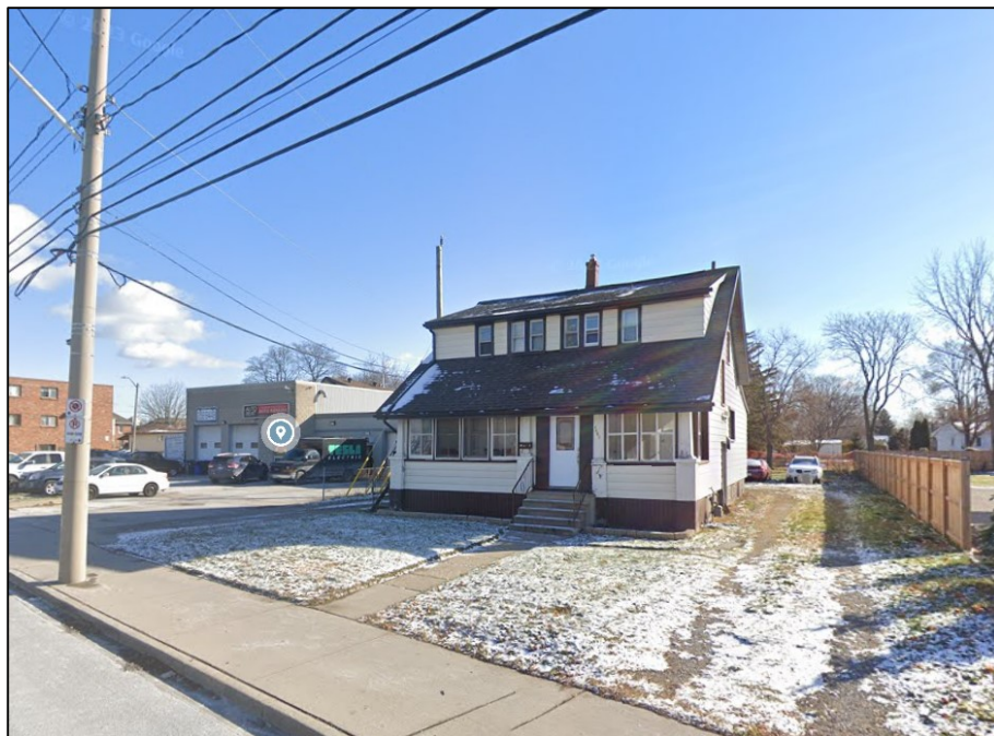
Figure 2 - Looking southeast towards 4461 Wyandotte Street East
