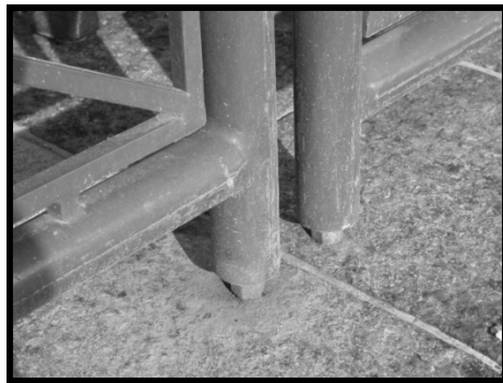
Upgraded surface treatment within Sidewalk Café.
