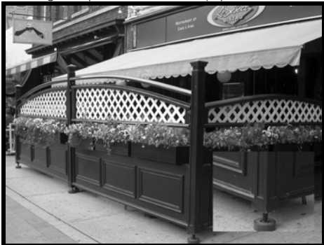
Alternative post attachment with no direct anchoring
