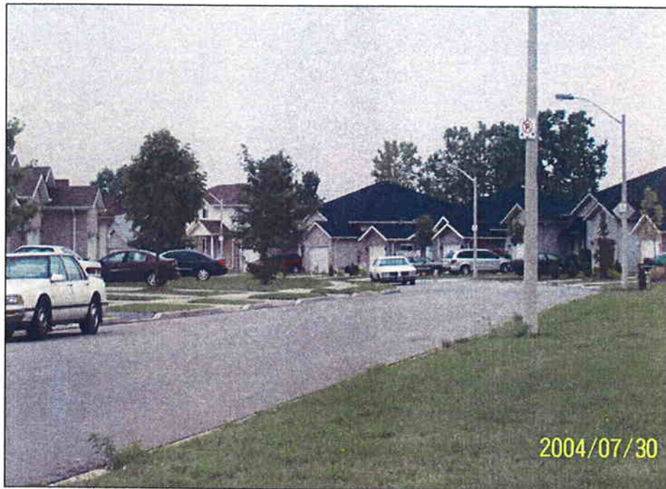
Photo 12- Looking North on Holburn Street
