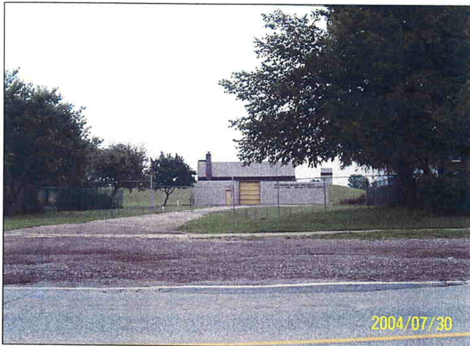
Photo 2- J.F. Cook Reservoir and Pumping Station
