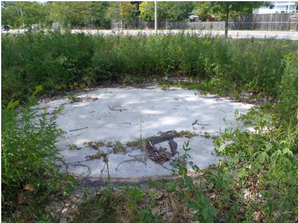
Plate B4: Site conditions showing concrete pad for structure; looking north
