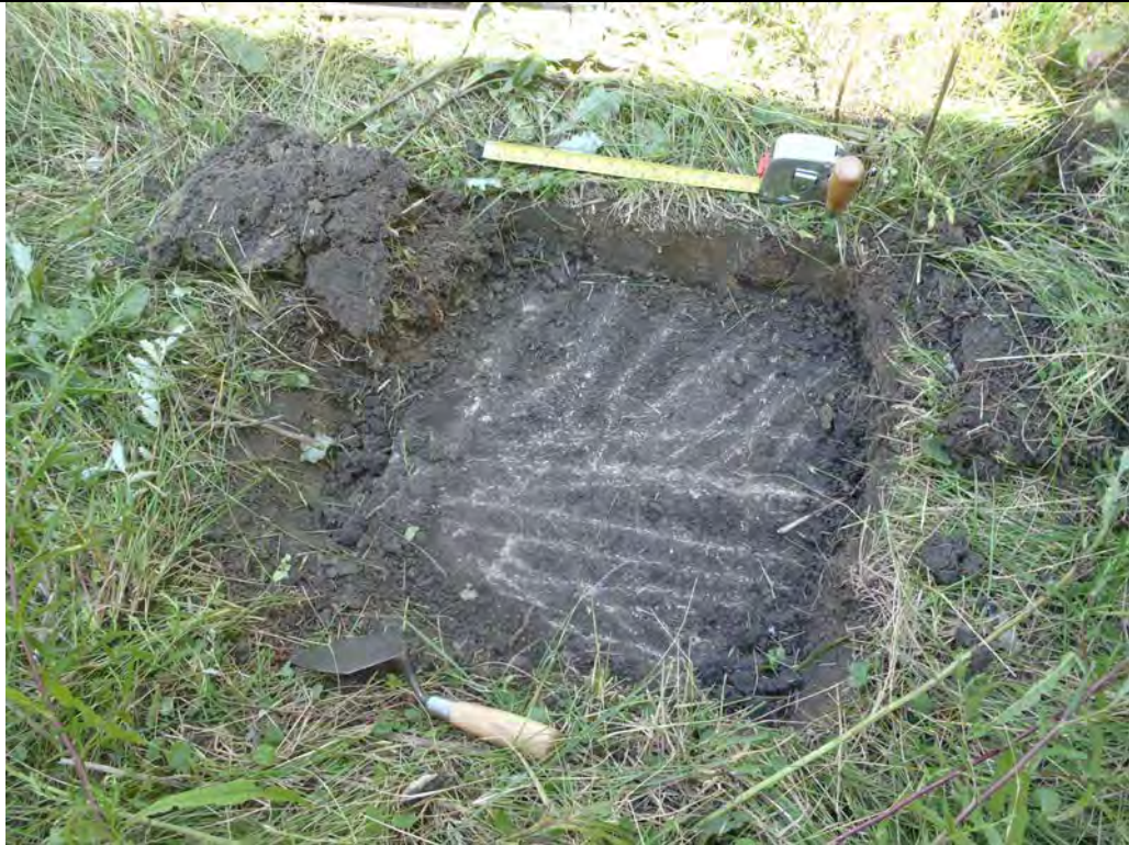
Plate B17: Test Pit showing concrete pad (Lot 8); looking east
