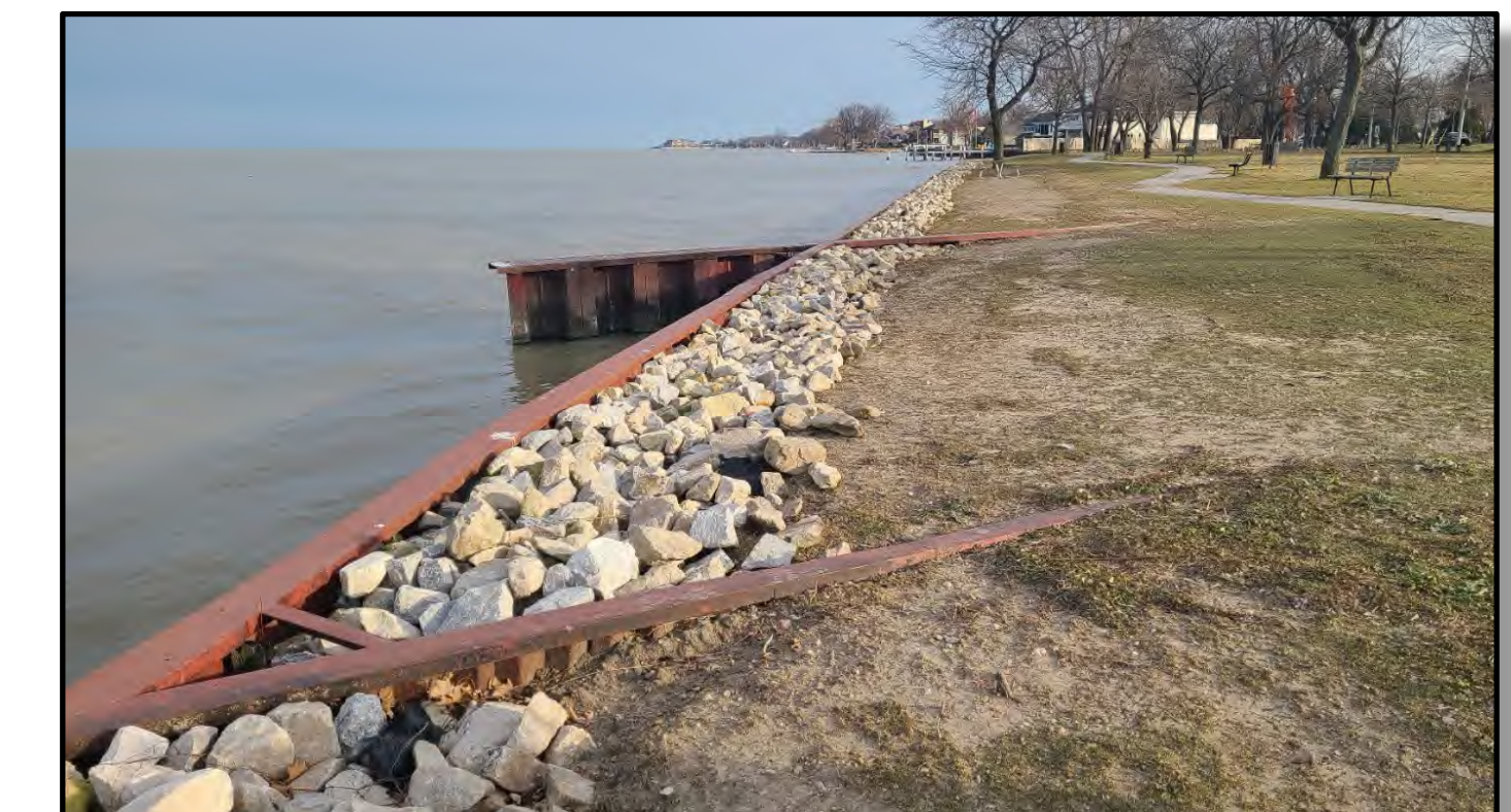
STEEL SHEET PILE SHORE WALL WITH ROCK APRON
