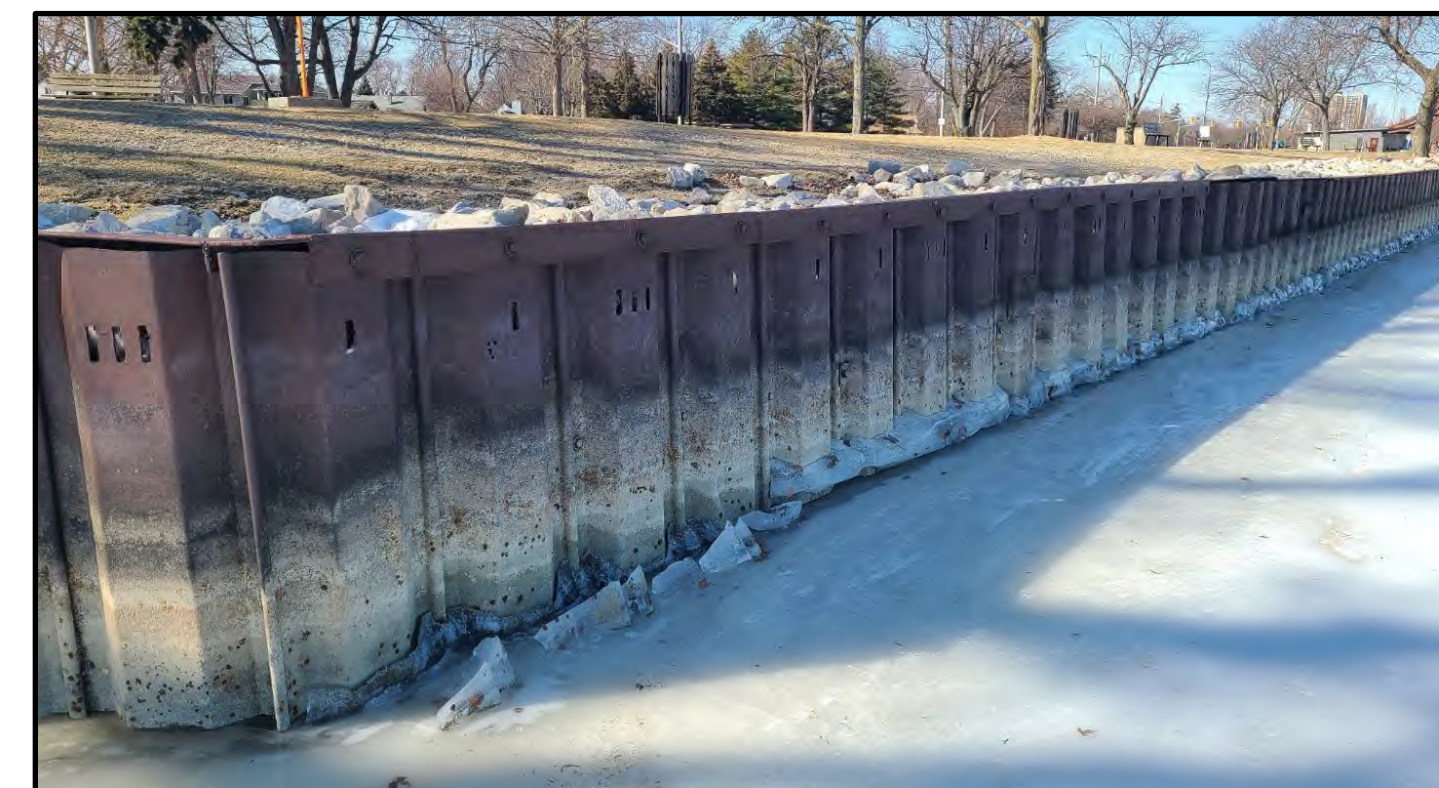
STEEL SHEET PILE SHOREWALL (SSP)
