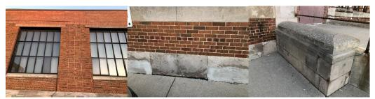
(Left) Cracking of masonry at gymnasium; (Right) Typical sections of stone/brick at base needing replacement/repair, and cleaning.
