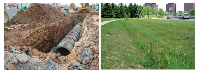
Figure 2: Storm Sewer Network (L) and Open Drain (R) Sample Images
