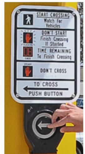
A raised (tactile) arrow is required on the pushbutton and provides information to pedestrians who are blind or low vision about which crosswalk is controlled by the pushbutton. It points in the direction of travel on the crosswalk and it is important for this to be aligned properly to assist blind and visually impaired pedestrians.
