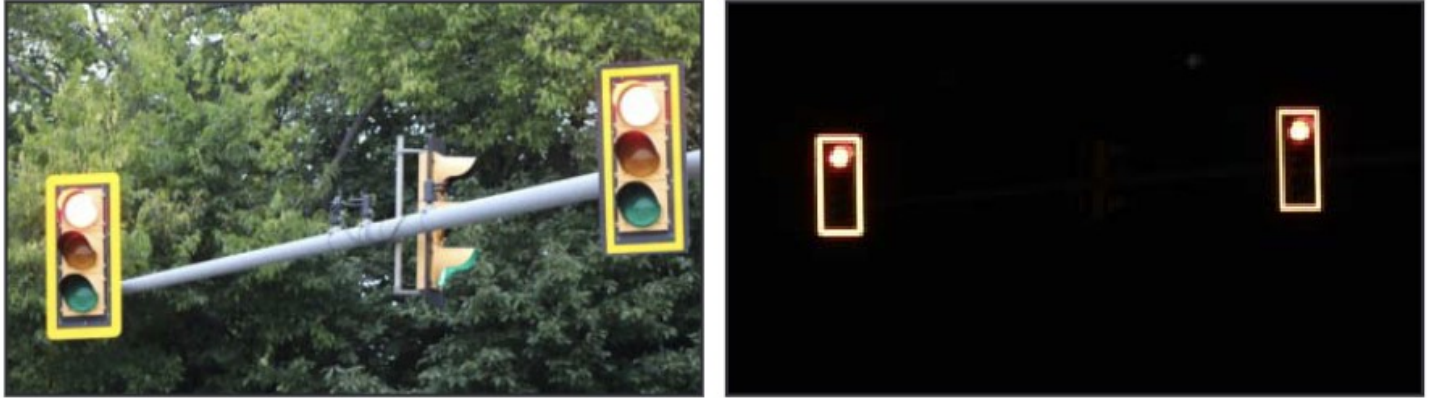
Figure 1: Retroreflective Backboards (source: Virginia DOT / FHWA)
