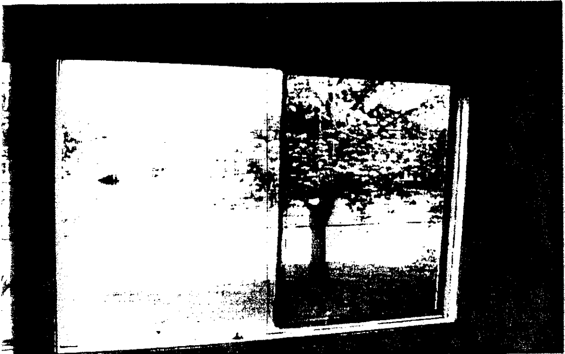
Photograph No. 7: North facing window of 2619, Suite No.15
