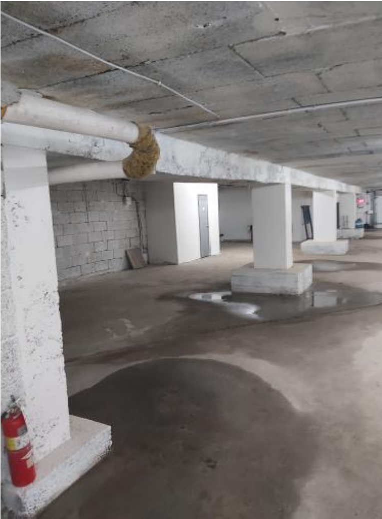
3. Condition of underground parking garage.
