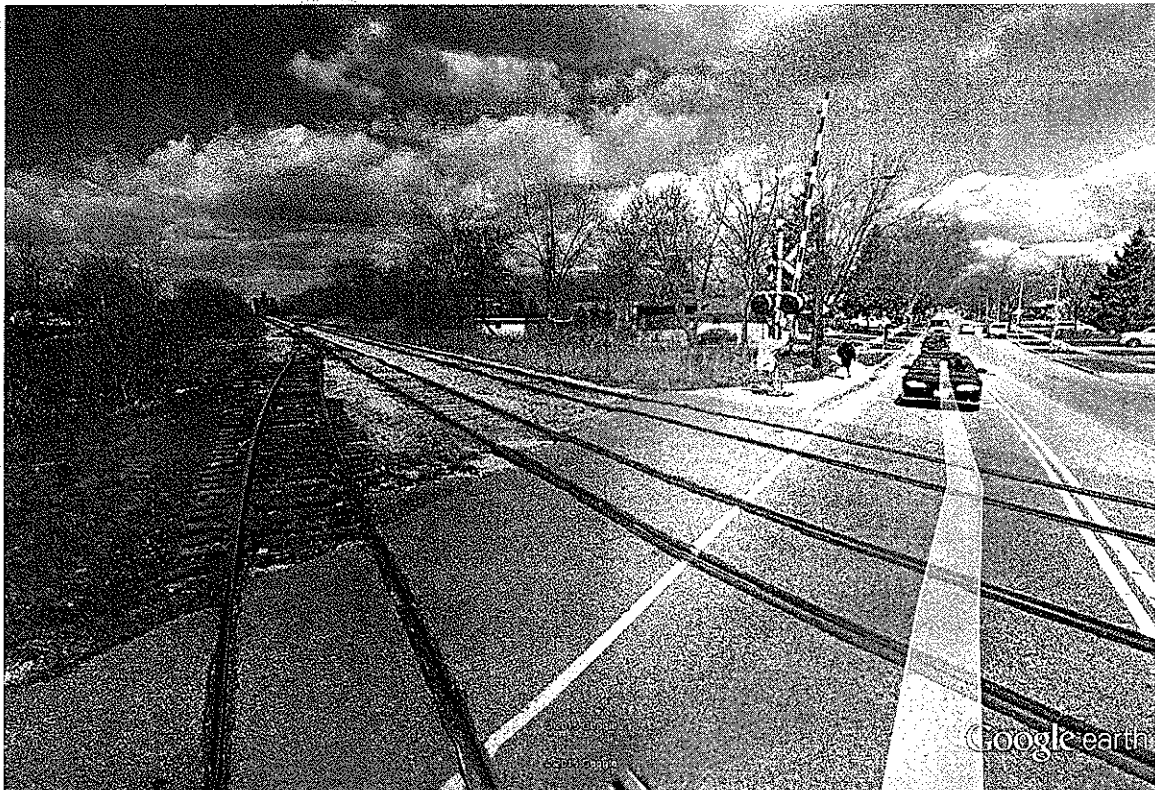
Figure 8: Grade Crossing Looking West
