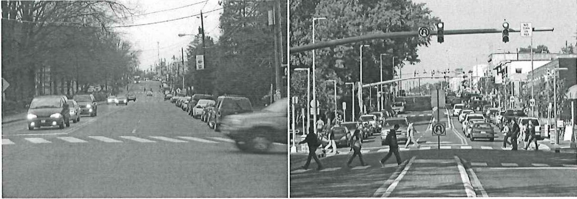
Hillsborough Street before and after reconstruction
