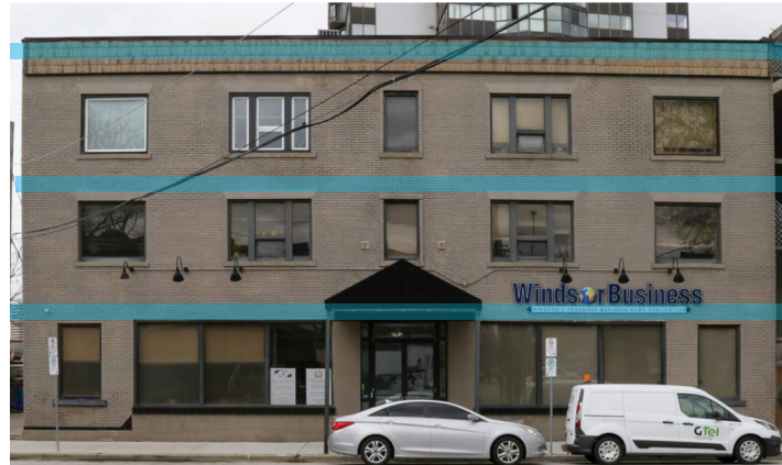
552 PITT STREET WEST
