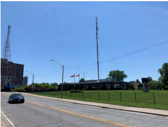
Plate 7: Looking south at CBC facility
