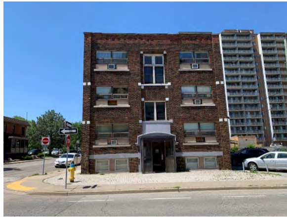
Plate 10: Looking west at Edwardian style apartment at 147 Janette Avenue
