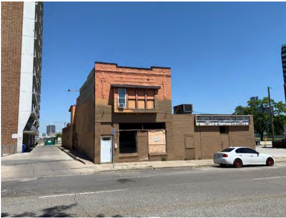
Plate 9: Looking north at commercial building at 656 Pitt Street
