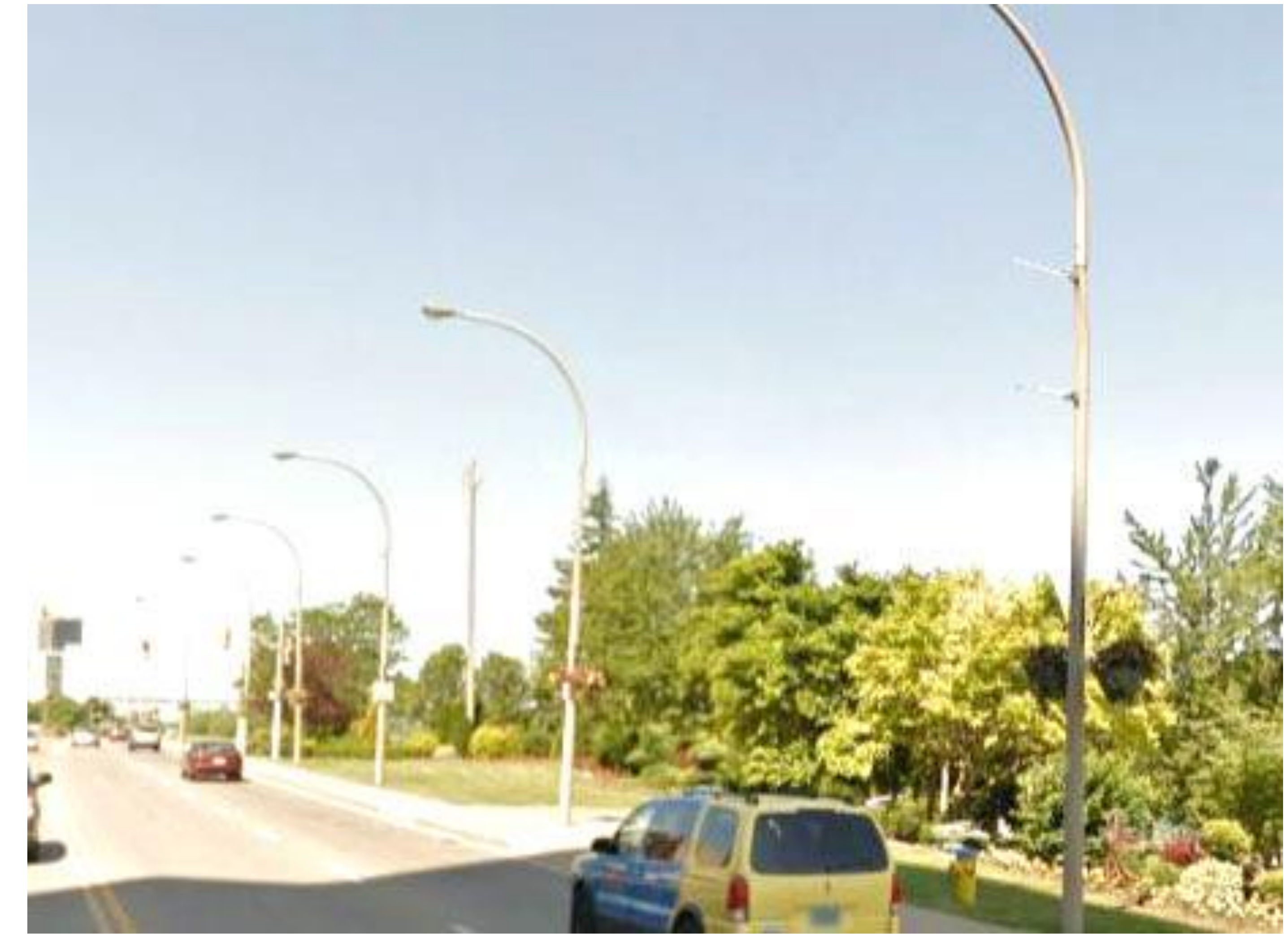
CONDITION 1 - CURRENT RIVERSIDE DRIVE STREET LIGHTS
