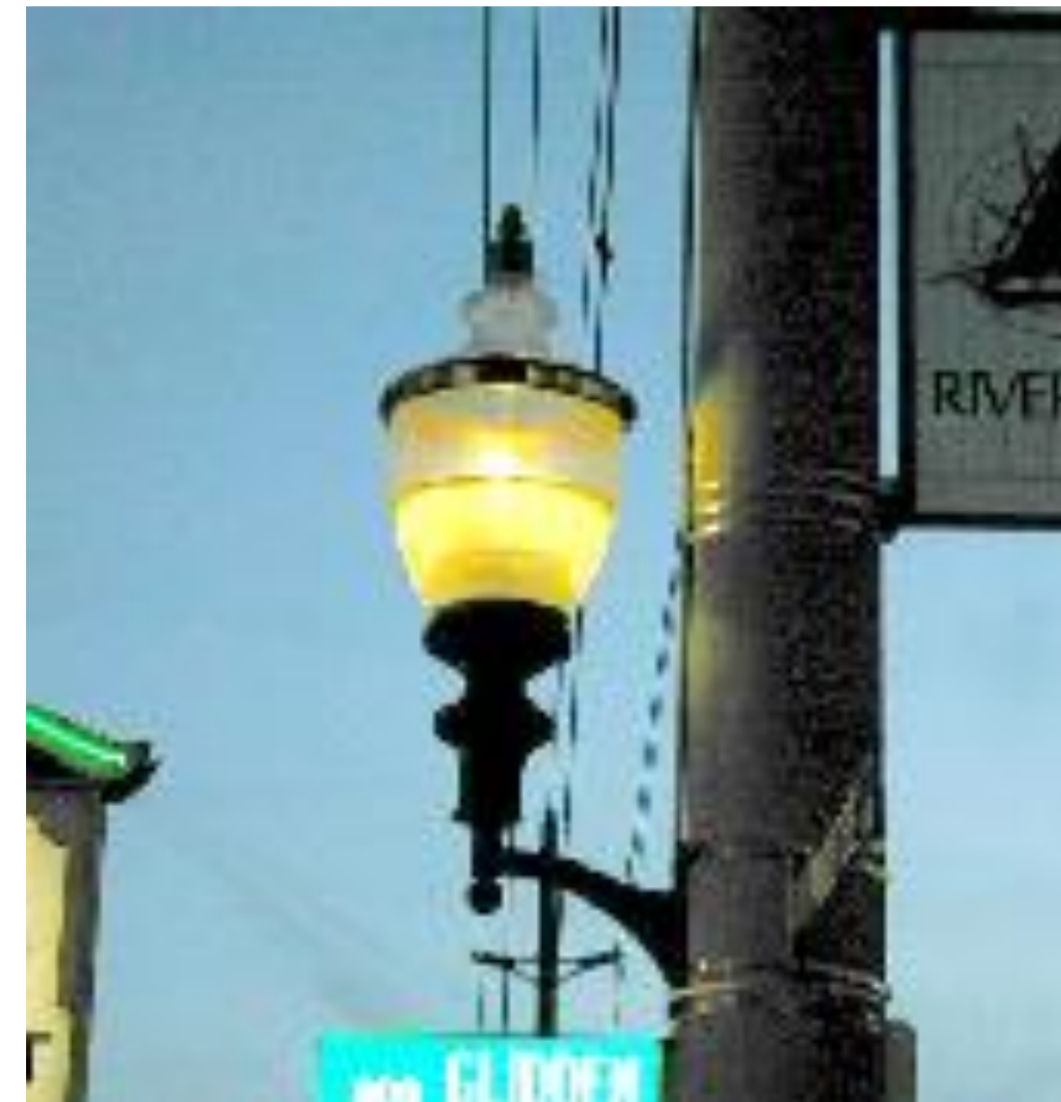
PEDESTRIAN FIXTURE MOUNTED ON STREET LIGHT STANDARD
