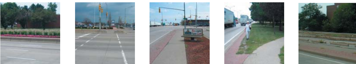
PEDESTRIAN AMENITIES ARE NOT ADEQUATELY PROVIDED
