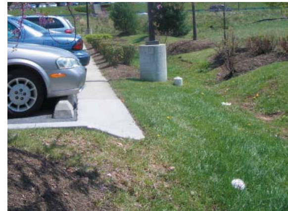
Bio-swales adjacent to parking lot
