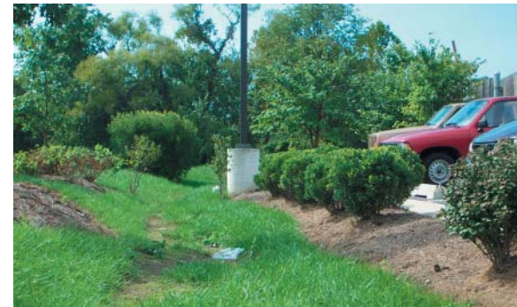
Bio-swales capture runoff from asphalted areas
